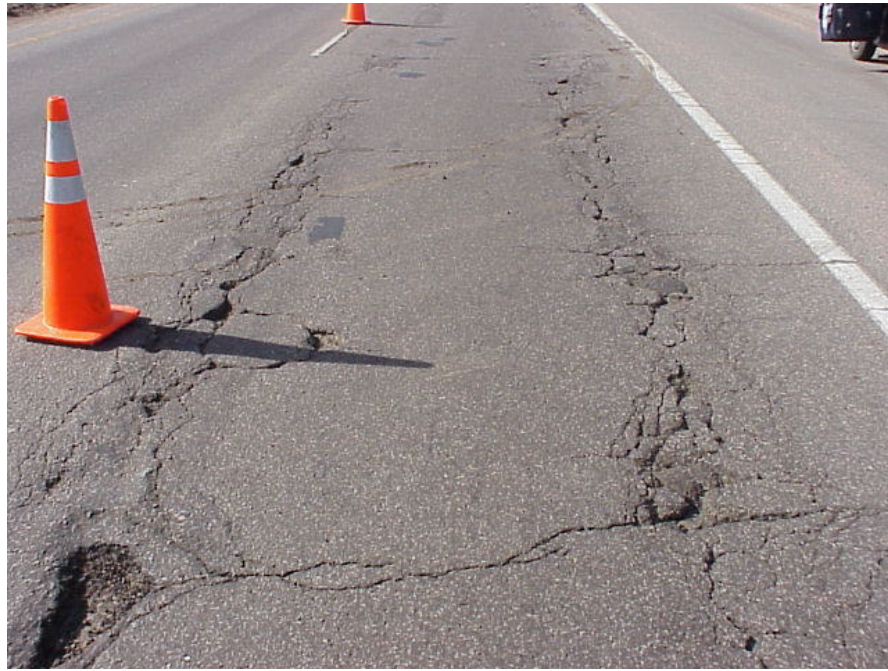
FIGURE 2. FATIGUE CRACKING OF TEST SECTIONS 1 AND 2
