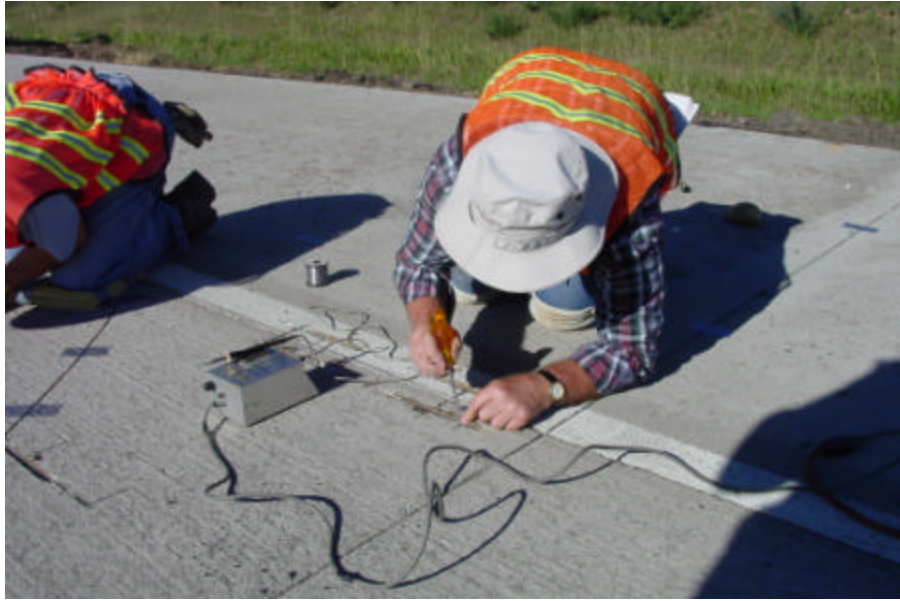
Figure 25. Soldering Leads to Installed Surface Gages
