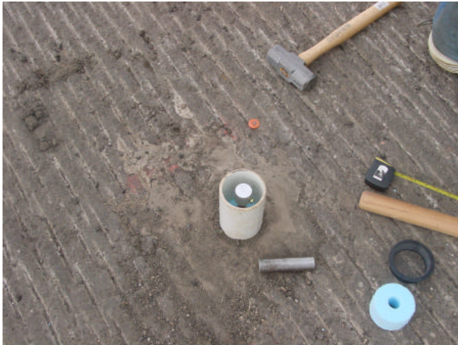
Figure 17. Installation of Reference Rods, continued
