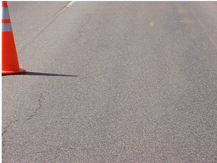
FIGURE 2. FATIGUE CRACKING OF TEST SECTIONS 1 AND 2
