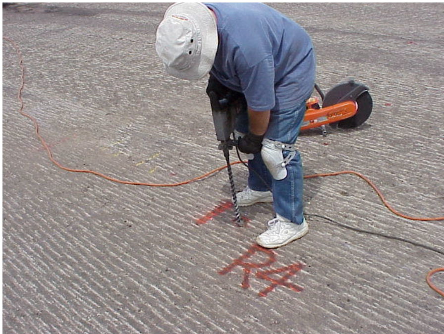
(b) Drilling holes into asphalt layer for embedded concrete gage installation
