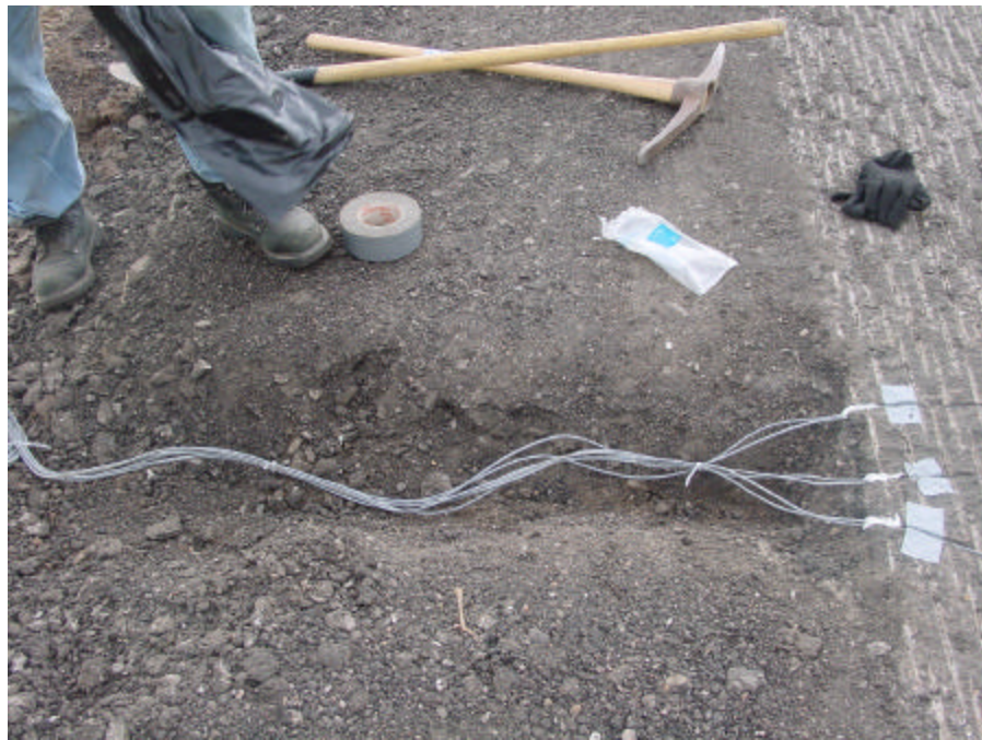
Figure 15. Recess and Protection of Lead Wires
