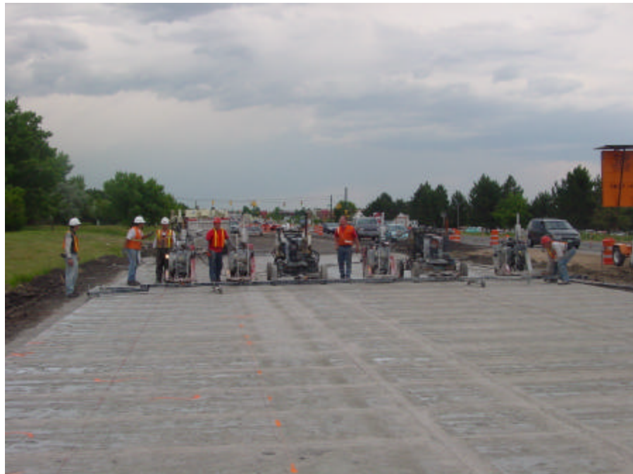
Figure 36. Sawing Transverse Control Joints
