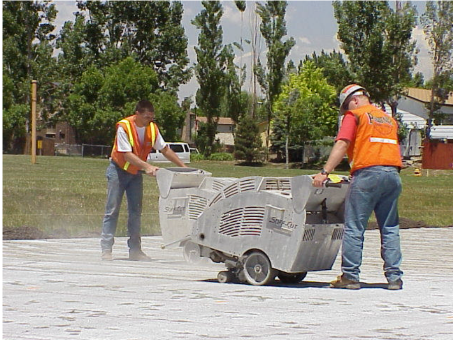
Figure 36. Sawing Transverse Control Joints
