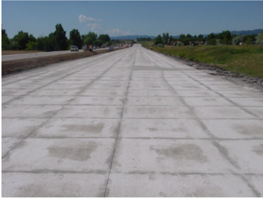
Figure 38. Pavement Surface After Joint Sawing
