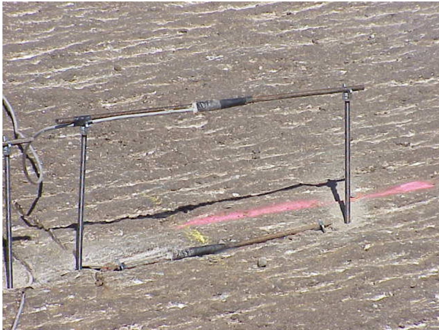
Figure 13. Installation of Embedded Strain Gages
