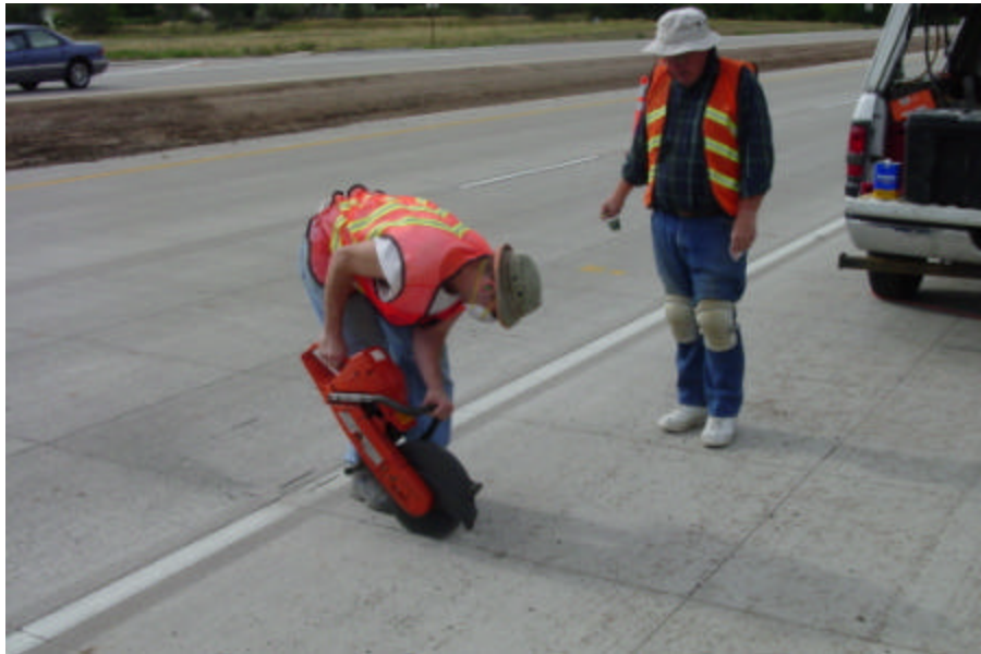
Figure 24. Cutting Grooves Along Joints for Gage Cables
