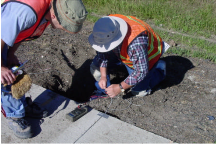
Figure 27. Checking Installed Gages
