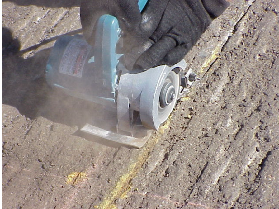
(a) Cutting groove using a diamond grinder
