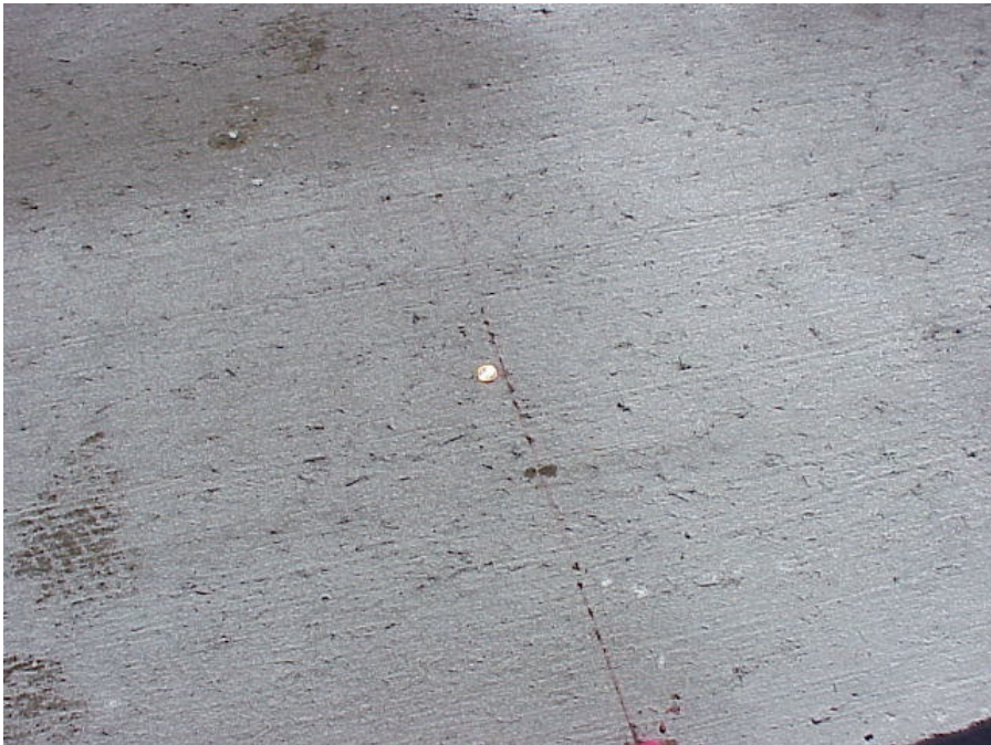
Figure 35. Surface Texture Provided by Astro turf Drag
