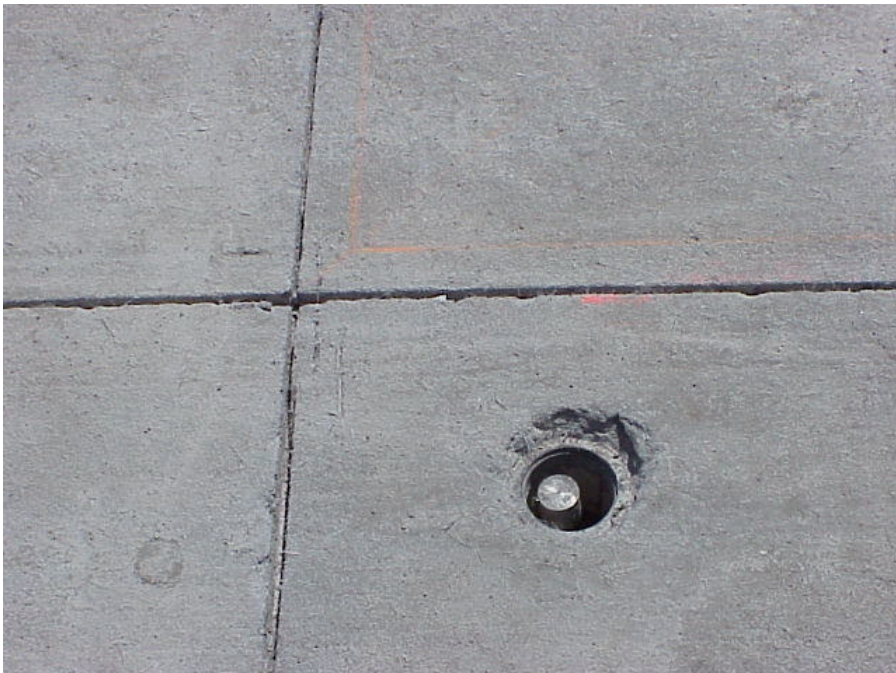
Figure 38. Pavement Surface After Joint Sawing
