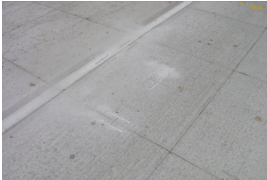
Figure 22. Recessed Slots on Concrete Surface for Gage Installation
