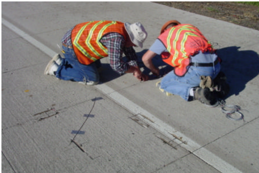
Figure 26. Recessing Leads
