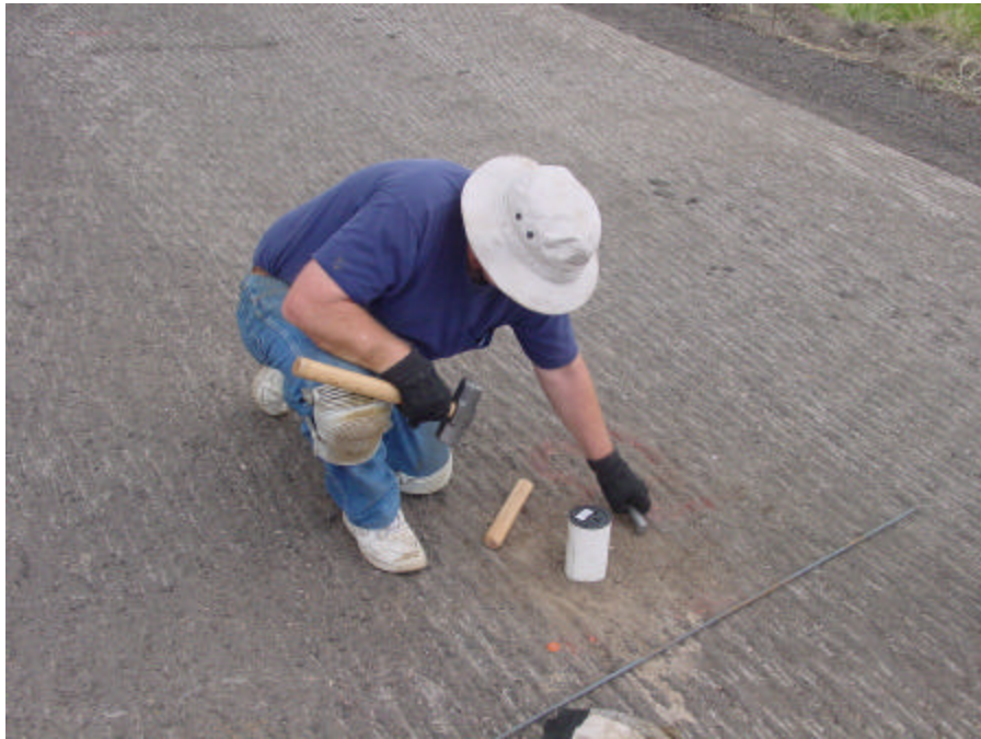
Figure 18. Completed Reference Rod Installation
