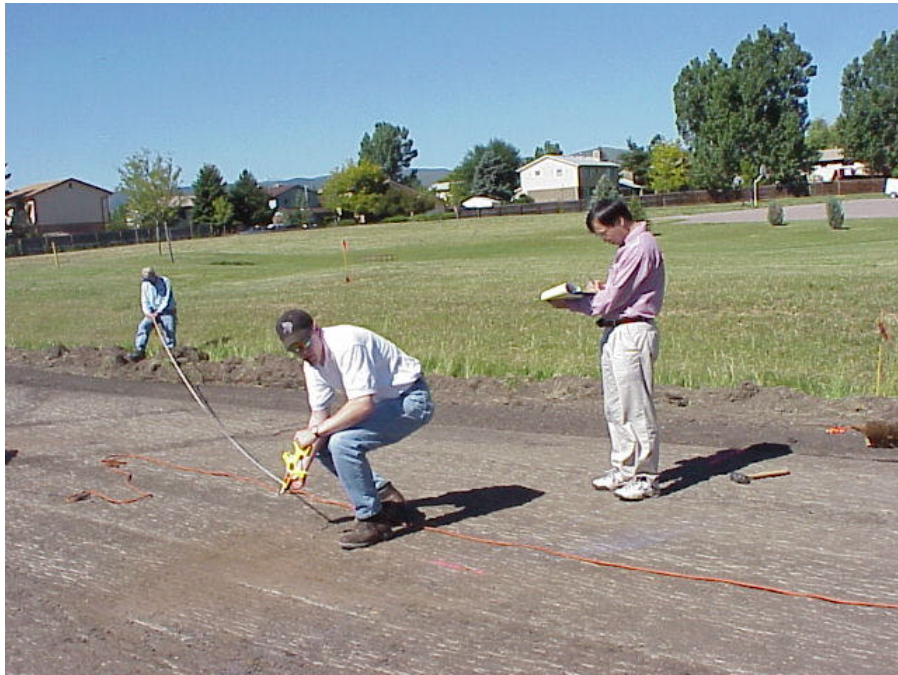
Figure 11 Setting Up Reference Points for Slab and Gage Locations
