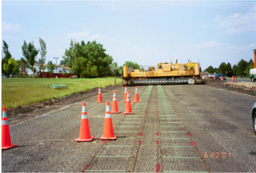
Figure 33. Tie Bar Assembly for Test Section 1
