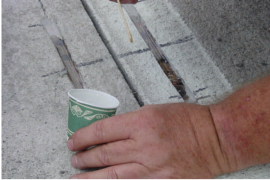
Figure 23. Attaching Strain Gages using Fast-Setting Epoxy
