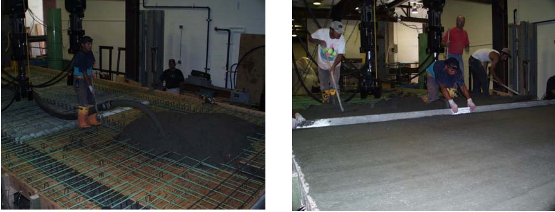
Figure 5.7 – Casting of the Deck
