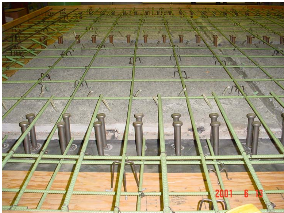
Figure 5.4 – Top Reinforcement
