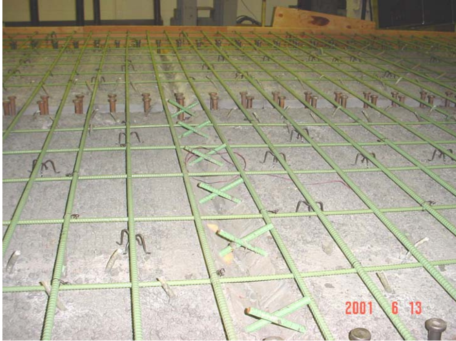
Figure 5.5 – Panel Splicing
