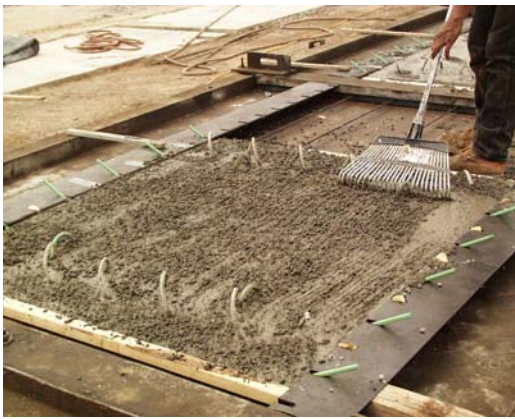
Surface Roughened with ¼-in amplitude
