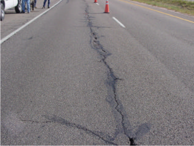
Reflective Cracking
