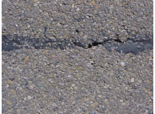
Top-Down Cracking
