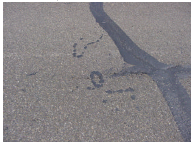
Reflective Cracking
