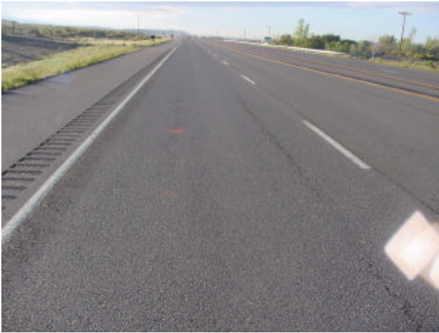
Top-Down Cracking
