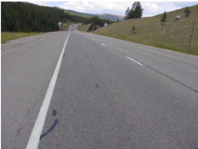
Top-Down Cracking
