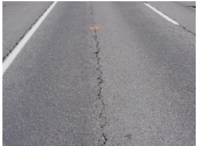
Top-Down Cracking
