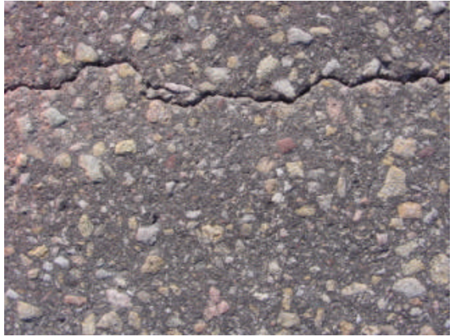
Top-Down Cracking
