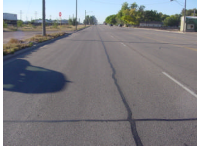
Top-Down Cracking
