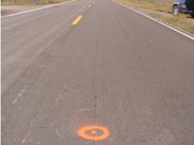
Reflective Cracking
