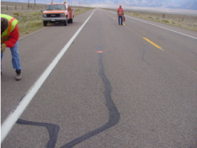
Top-Down Cracking
