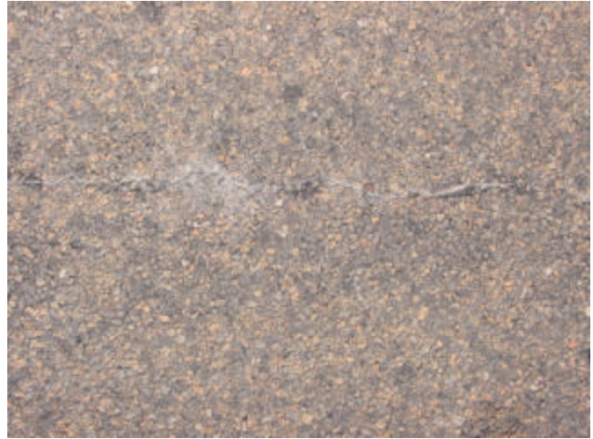
Reflective Cracking
