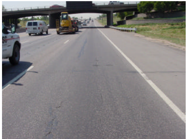
Top-Down Cracking
