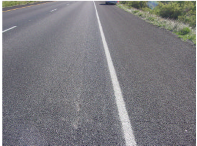
Top-Down Cracking
