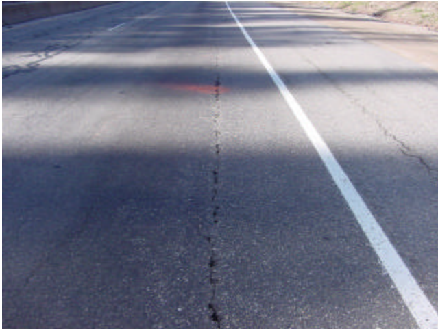
Top-Down Cracking
