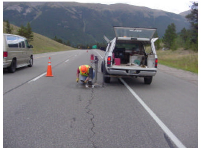
Top-Down Cracking
