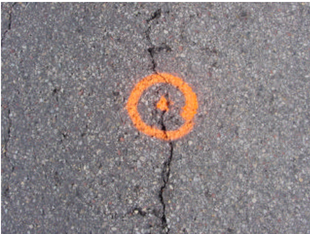
Top-Down Cracking
