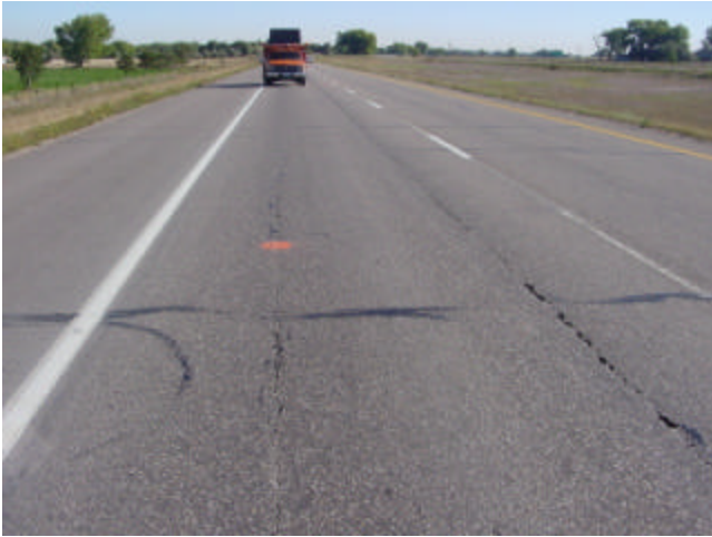
Top-Down Cracking
