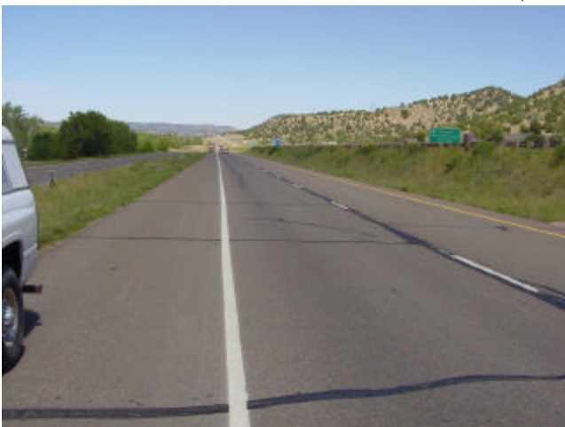
Reflective Cracking
