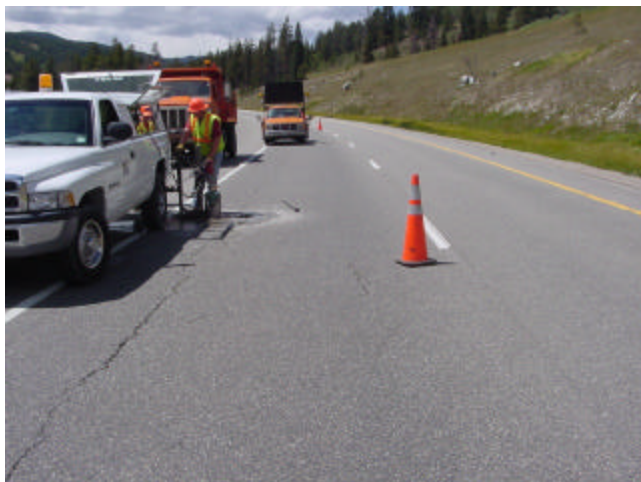
Top-Down Cracking
