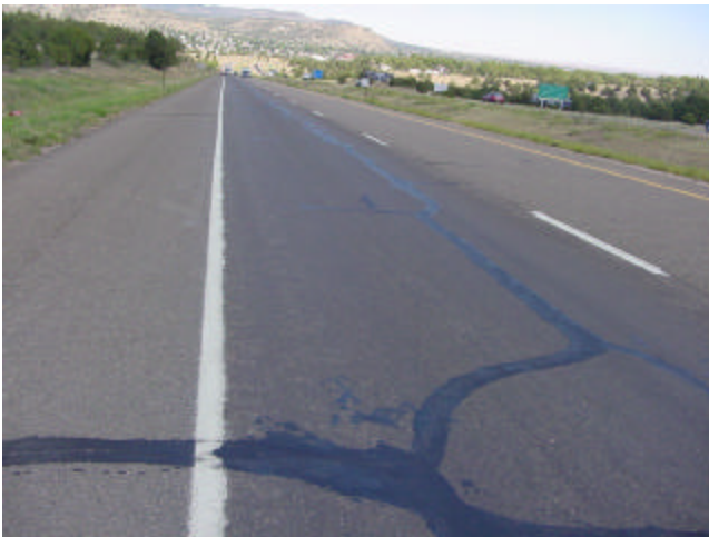
Reflective Cracking
