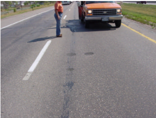
Top-Down Cracking
