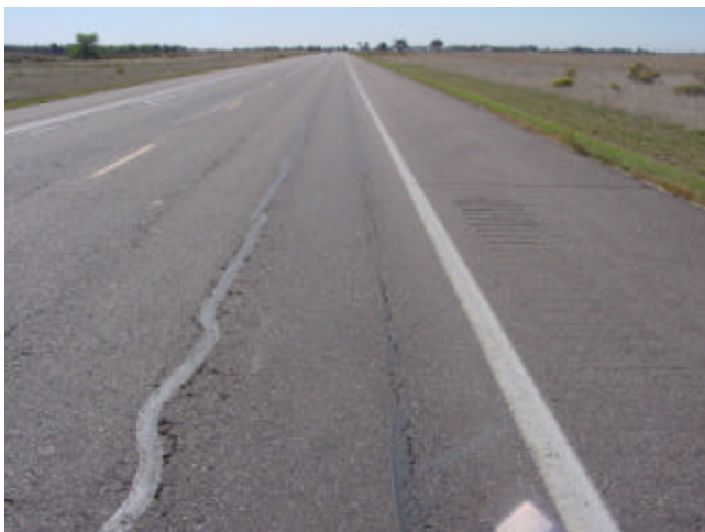
Top-Down Cracking
