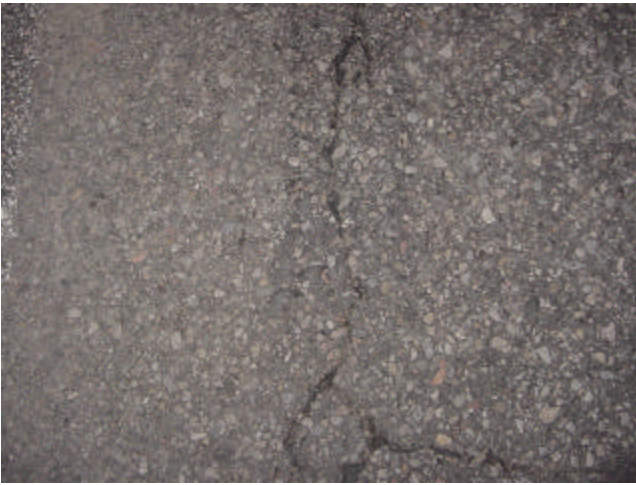
Reflective Cracking
