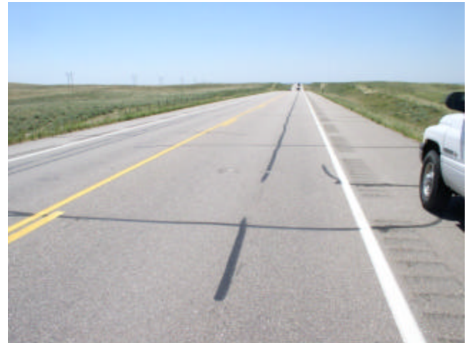
Reflective Cracking
