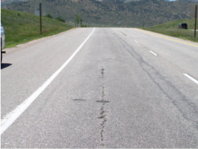
Top-Down Cracking
