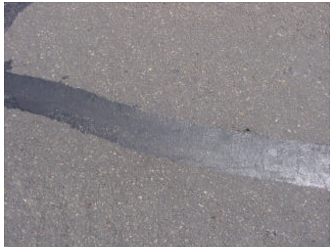
Reflective Cracking
