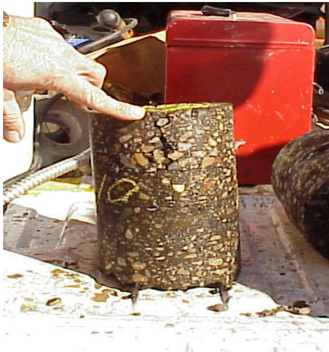
Figure 7. This crack is top-down as you can see it is only visible in the top lift
