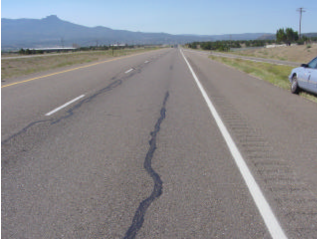
Top-Down Cracking
