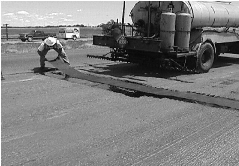
Figure 8 – Proguard placement.
