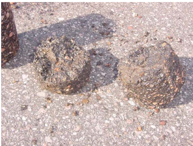
Figure 19 - Fragmented and badly stripped cores .
