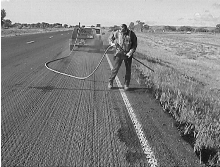
Figure 9 – Equipment used to clean cracks prior to filling with sealant.
