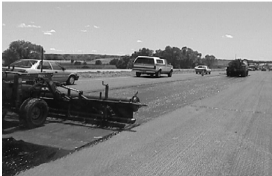
Figure 6 – Placement of Petromat material.
