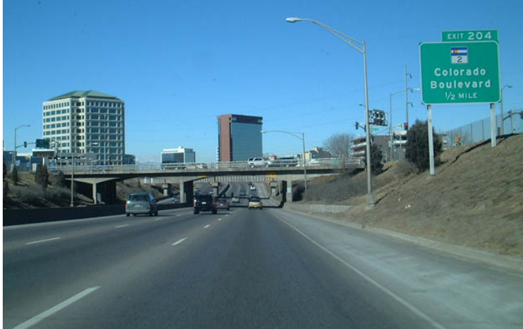
Figure B-2 Northbound Interstate 25 approaching Junction Colorado 2 (Colorado Boulevard), Exit 204
