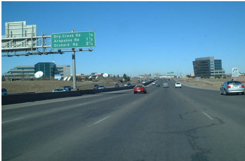
Figure B-3 Northbound Interstate 25 approaching Dry Creek Road (Exit 196)
