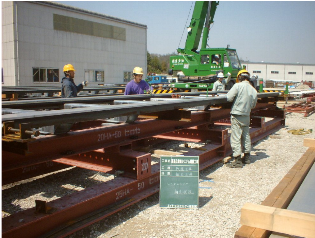
Figure 46: Levitation Rail Section Assembly Prior to Installation
