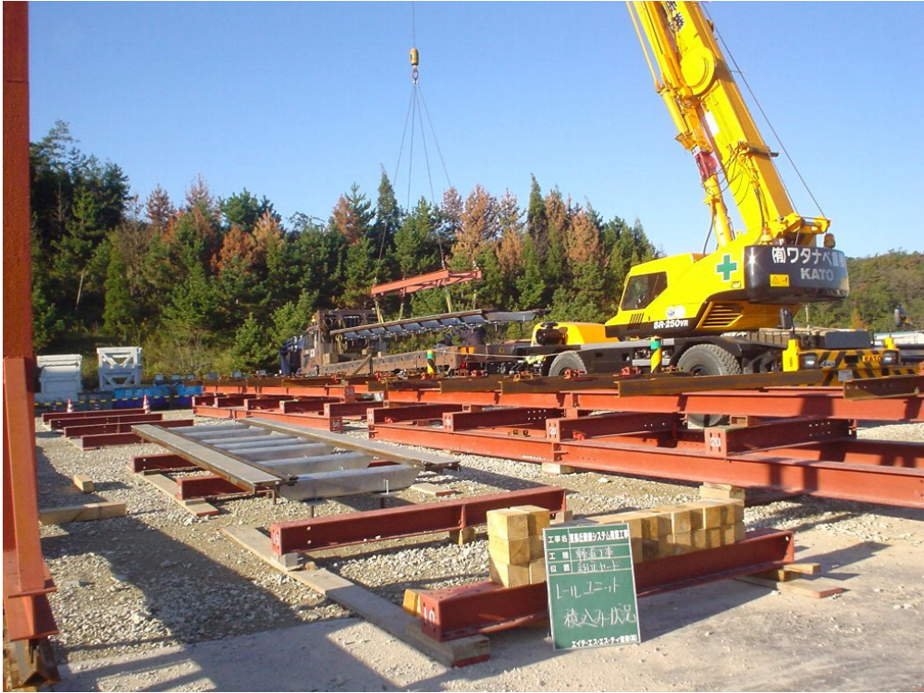
Figure 47: Guideway Section Staging for Transport Over the Guideway
