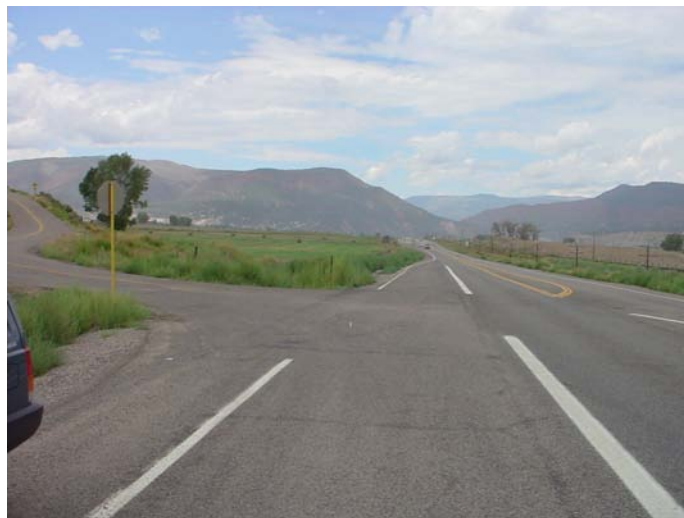
Figure 25: Eagle County Airport access roadway
