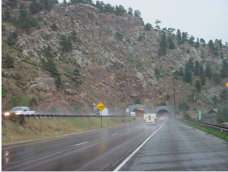
Figure 17: I-70 Eastbound at Twin Tunnels
