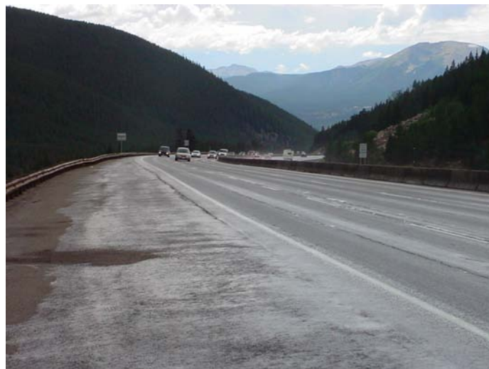
Figure 21: I-70 Westbound west of Eisenhower-Johnson Memorial Tunnel
