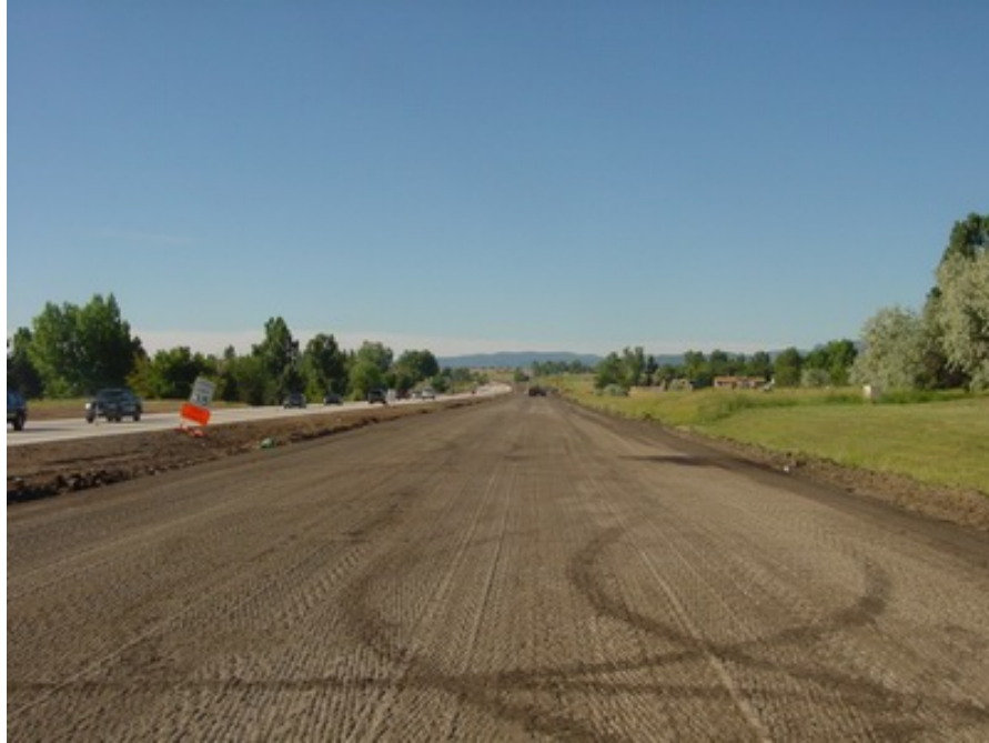
Figure C.1. Milled Surface of Existing Asphalt Pavement
