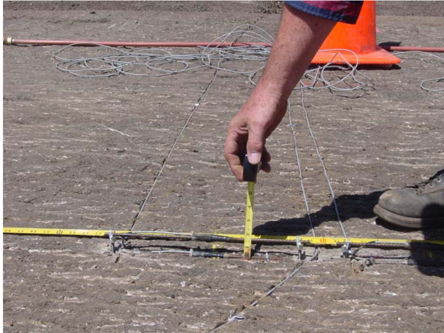
Figure D.4. Typical Embedded Strain Gage Installation
