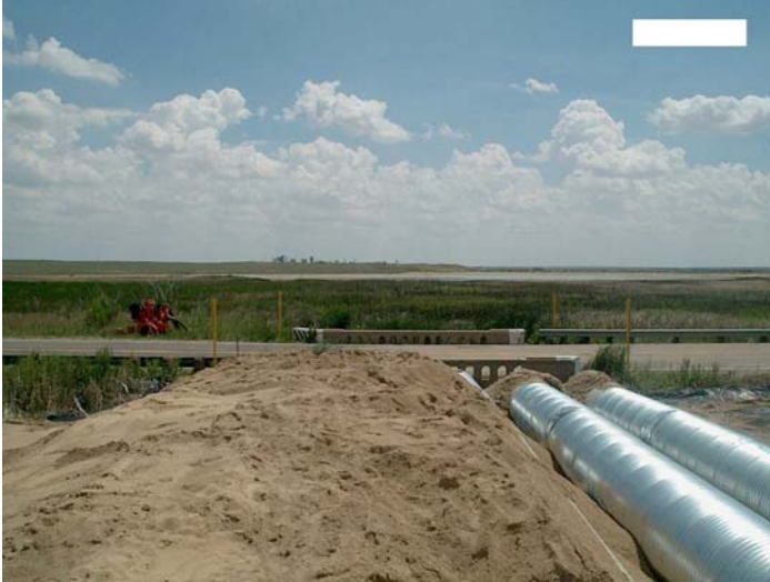
Figure 3.2. Construction of detour culverts on US Highway 50 by John Martin Reservoir in CDOT Region 2 within environmentally sensitive areas.
