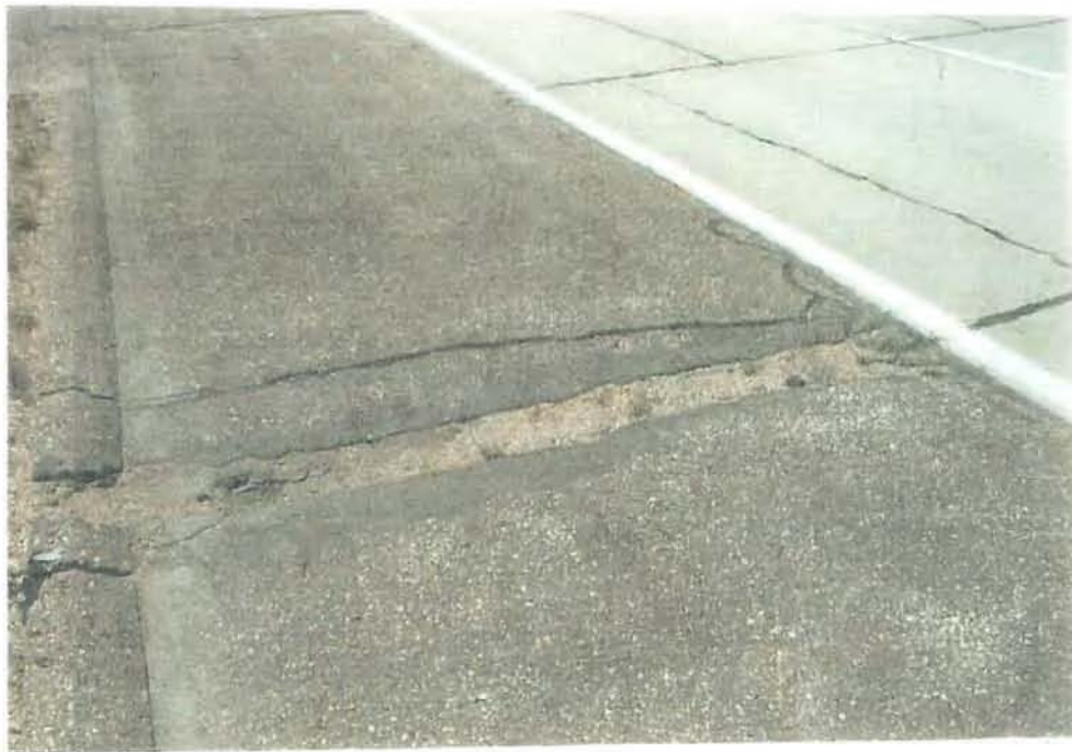
Figure 2. Pre-construction Roadway and Shoulder Condition
