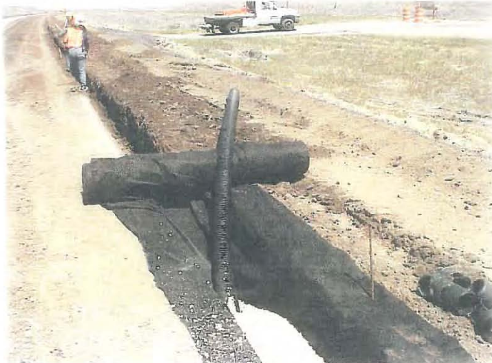
Figure 3. Typical Edge Drain Construction
