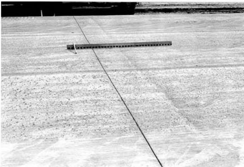
Photo 5: Transverse indentation of plastic concrete
