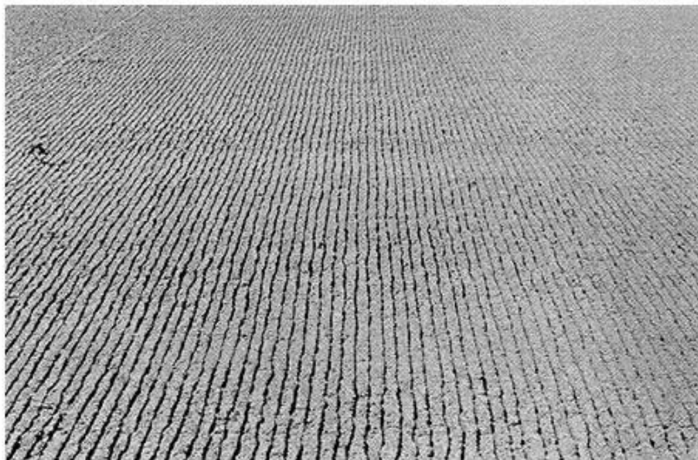
Photo 12: 1/2-inch uniform spaced transverse tining
