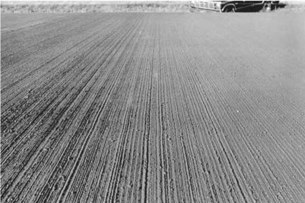
Photo 9: Close-up of transverse astro-turf texture
