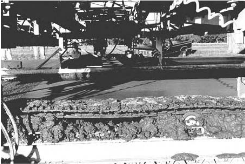
Photo 8: Installation of transverse astro-turf texture
