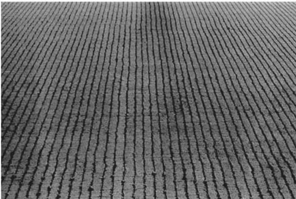
Photo 11: 1-inch uniform spaced transverse tining (state standard)
