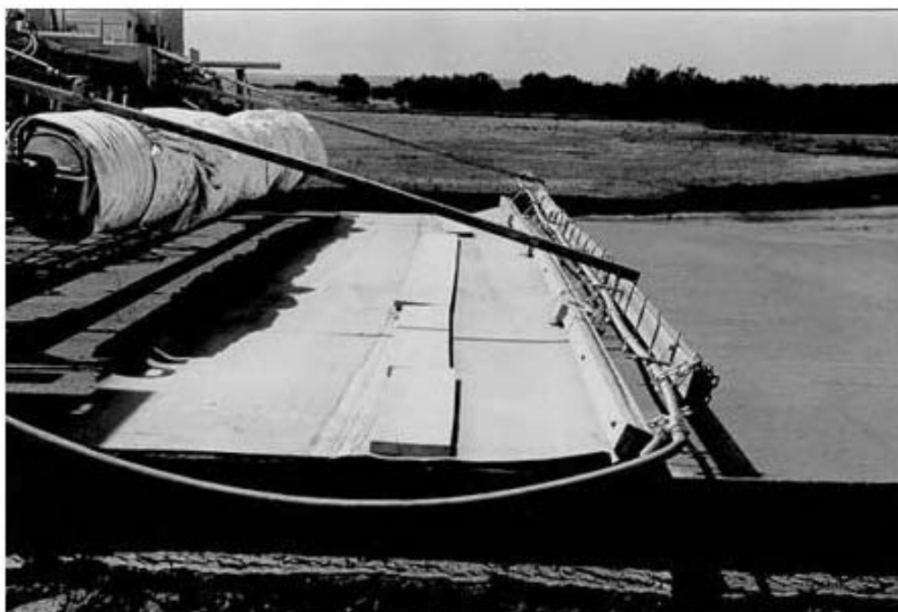
Photo 6: View of the astro-turf drag with planks for added weight
