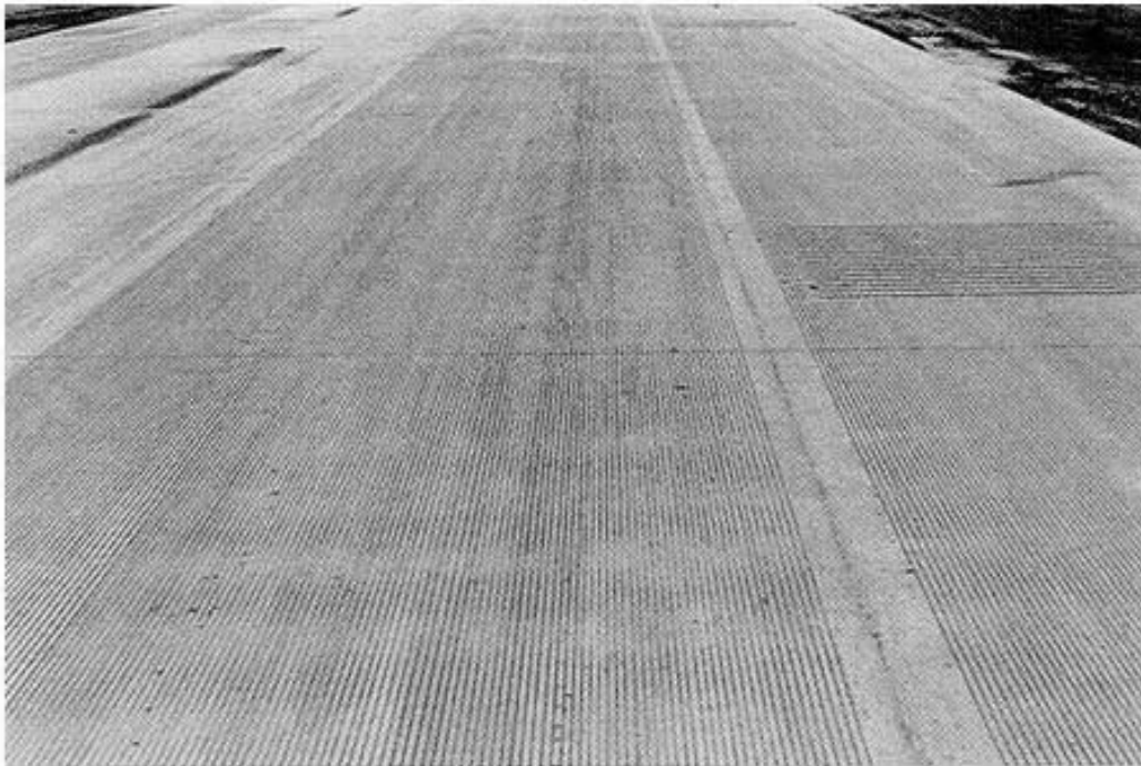
Photo 16: Grooved rumble strip in the right shoulder
