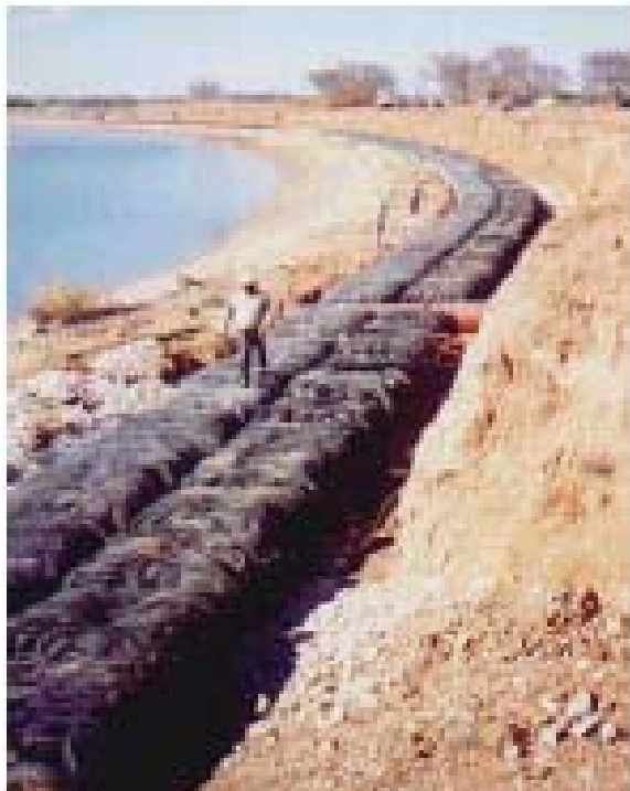
Figure A1. Tire Bales as Erosion Control (during construction)
