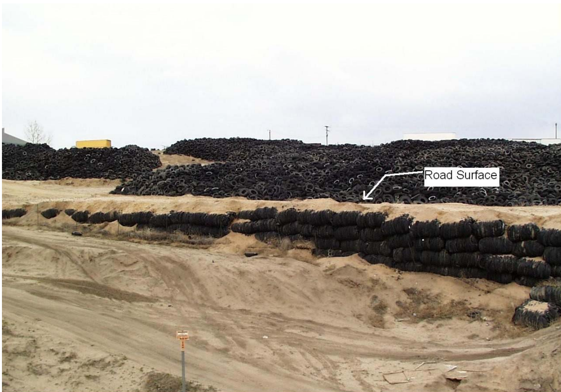
Figure B3. Road built from stacked tire bales.
