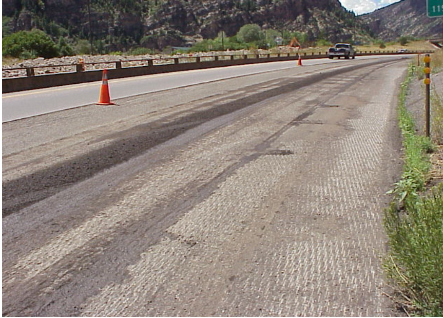
Figure 4. The Surface Was Planed to a Depth of 1-1/2 inch.
