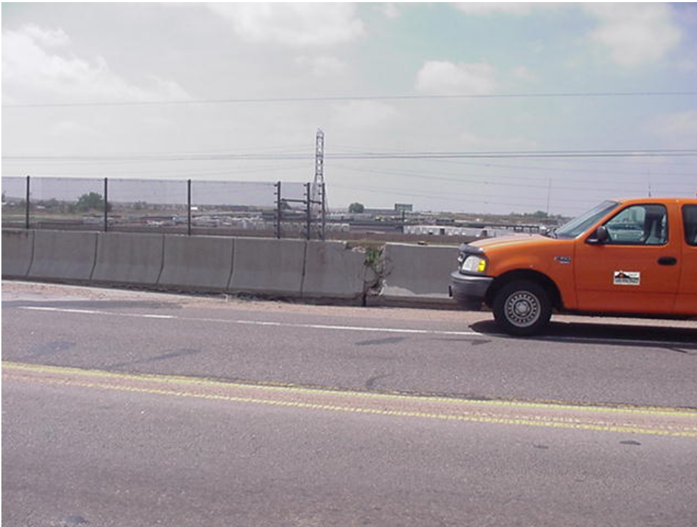
Figure C.10. Photos of Structure E-17-VR in Region 6
