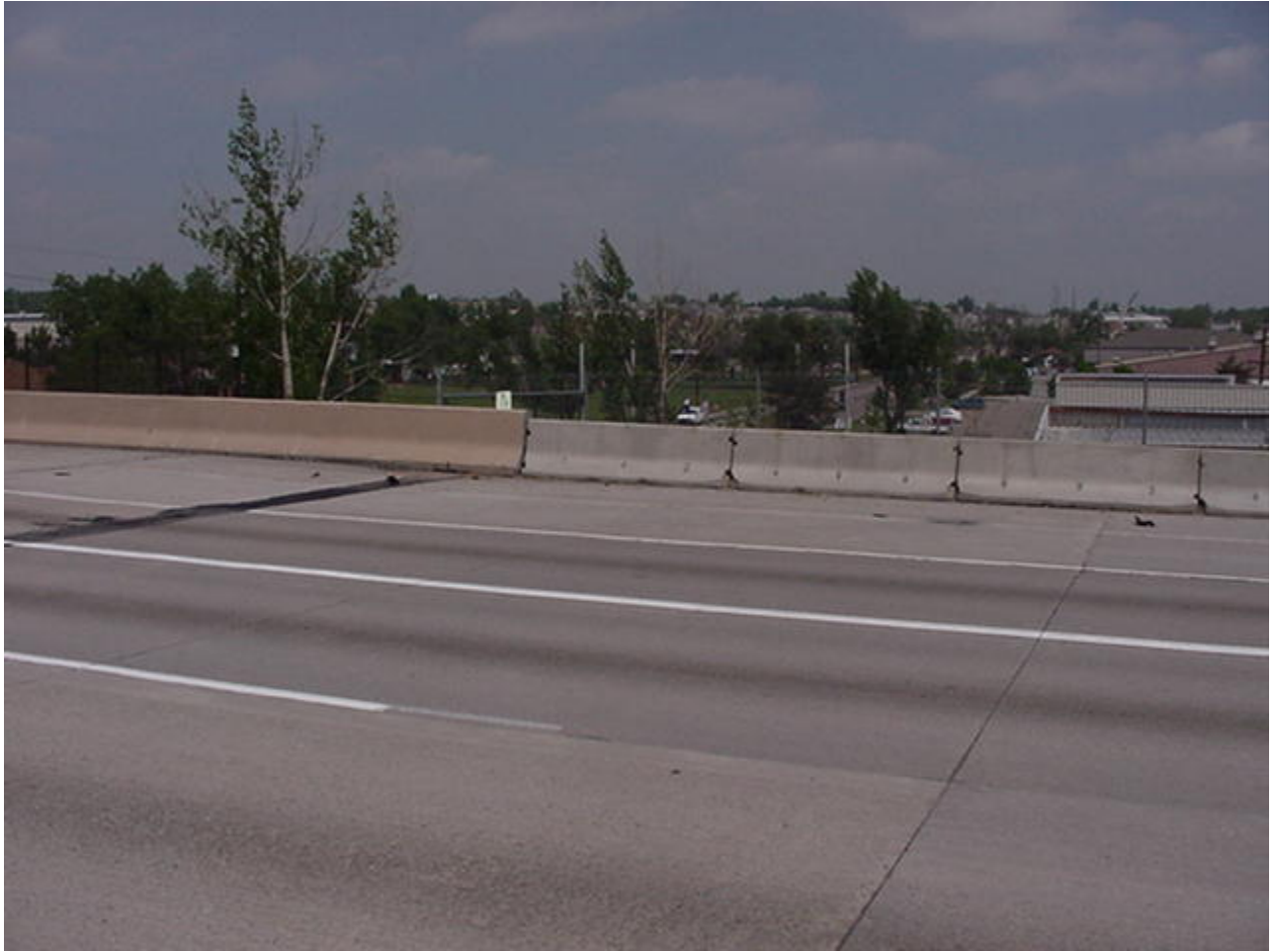
Figure C.12 Photo of Structure E-17-QA in Region 6
