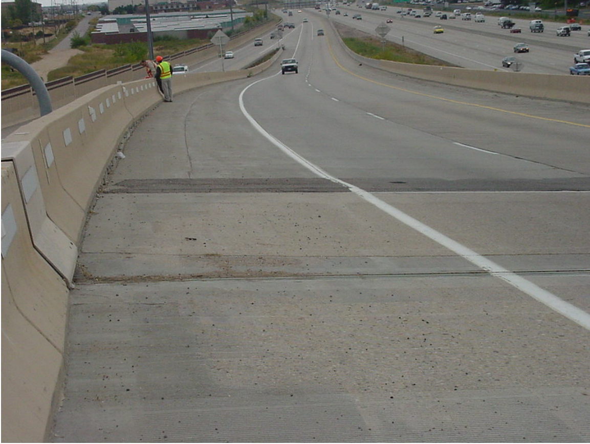
Figure C.4. The Eastern Side of the Bridge and Roadway Approaches of the I70/I-225 Interchange (Structure E-17-SW in Region 6).
