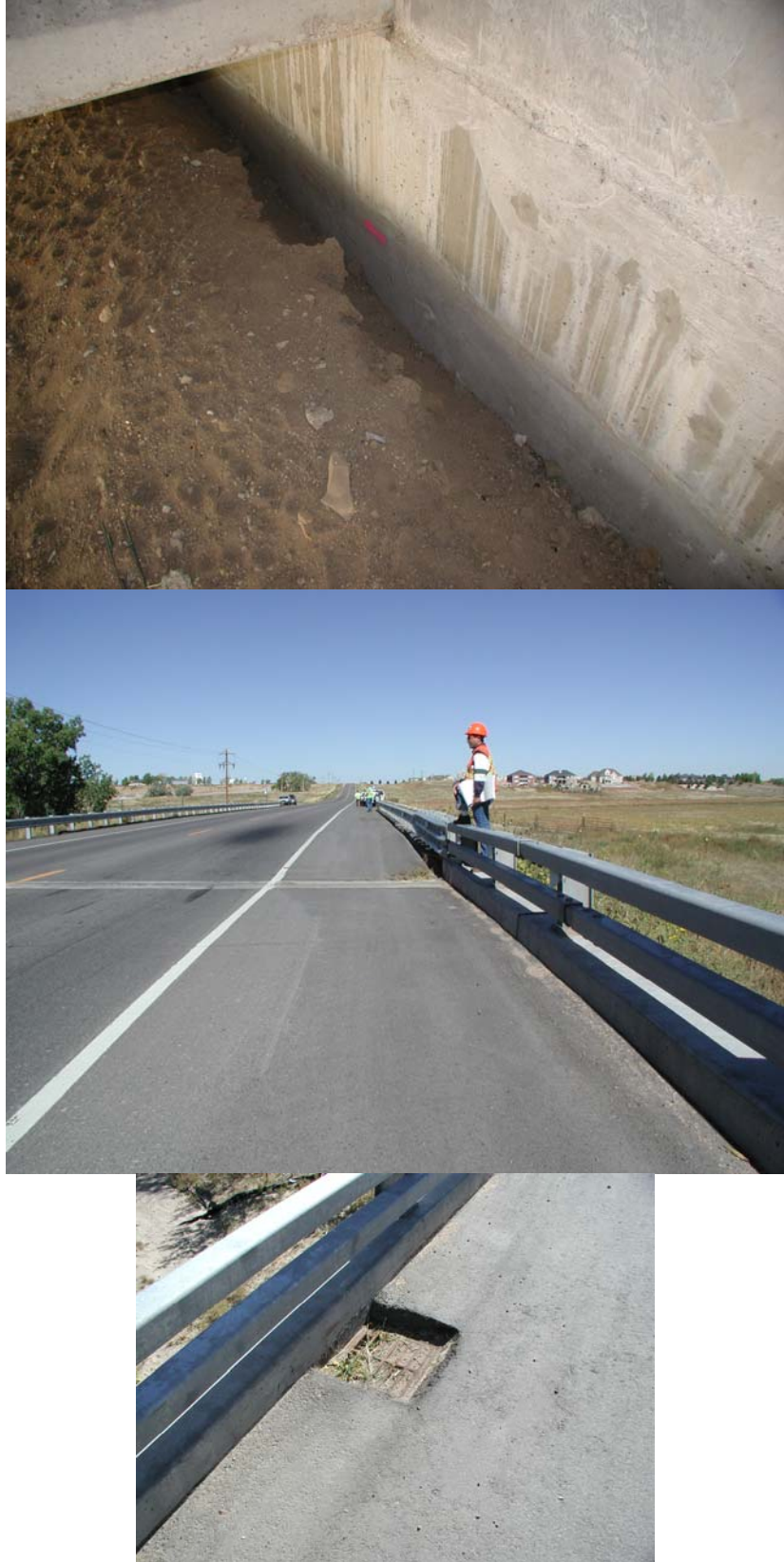
Figure C.15. Photos of Structure E-19-Z in Region 1 before Repair
