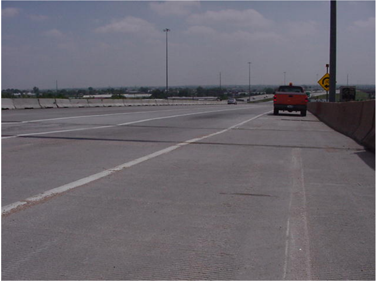
Figure C.11. Photo of Structure E-17-QA in Region 6
