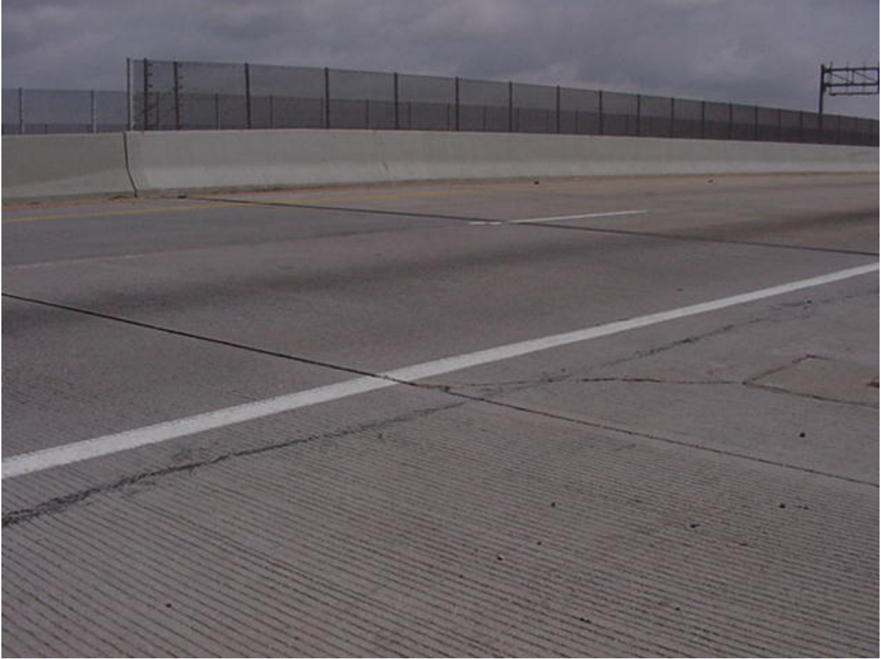
Figure C.9. Photo of Structure E-17-PS in Region 6
