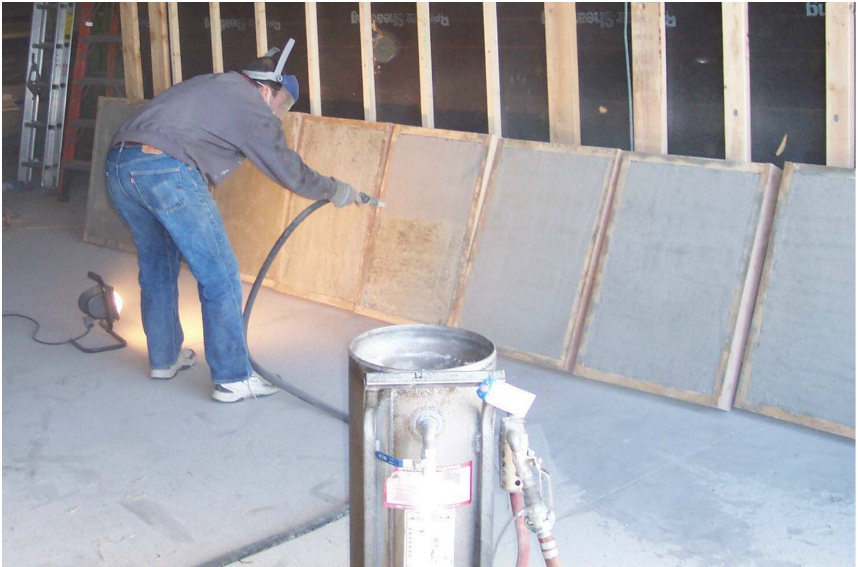
Sandblasting off the Liquid Curing compound at 14-days
