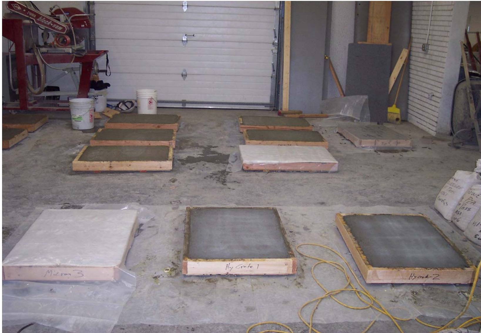
Test panels at the beginning of 14-day curing period.
