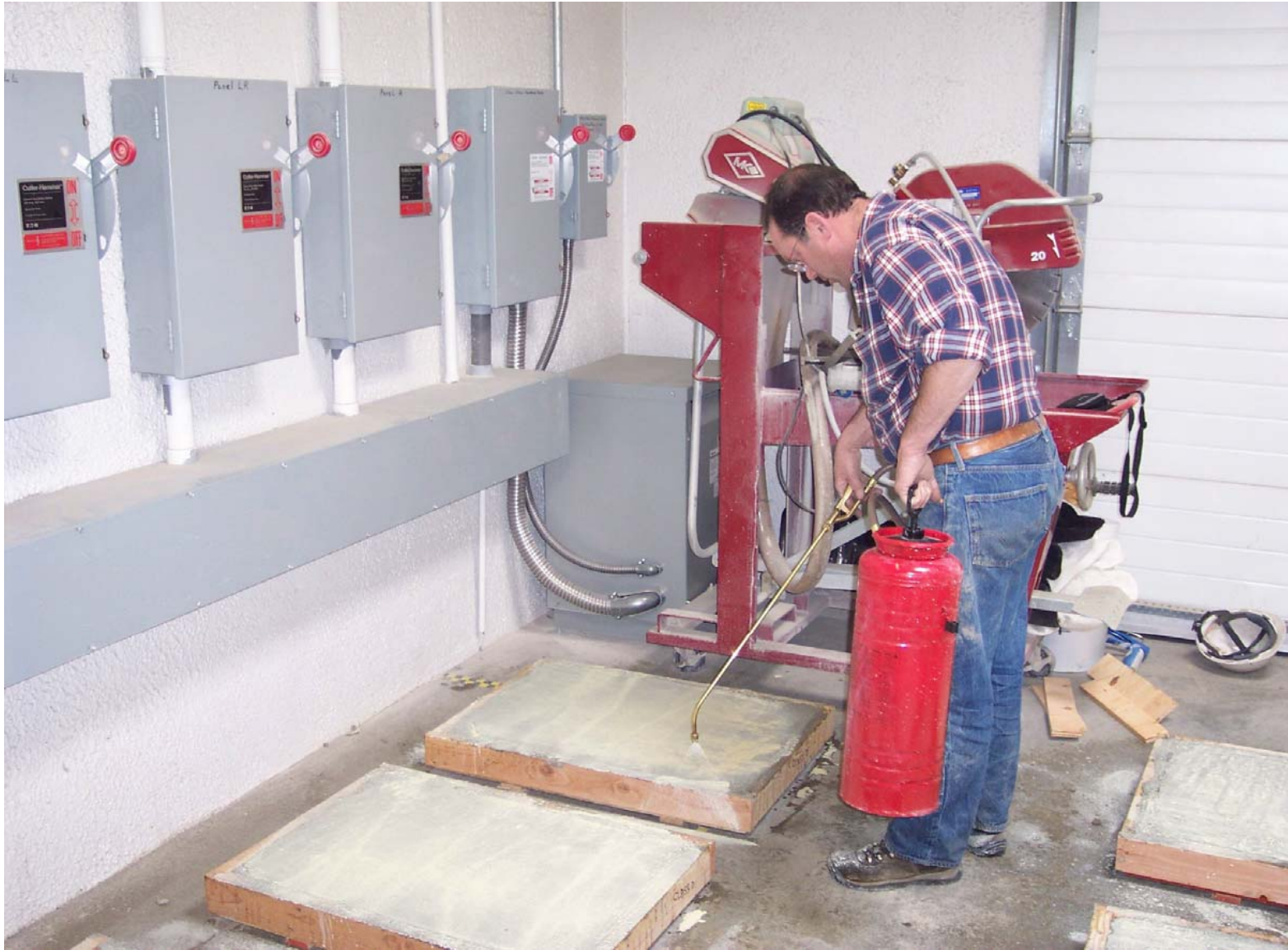
Application of CDOT-Approved Liquid Curing Compound to Most Panels
