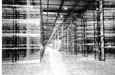
Concrete floors designed with joint spacing of 150-ft provide building owners with a very low life cycle cost floor solution.
