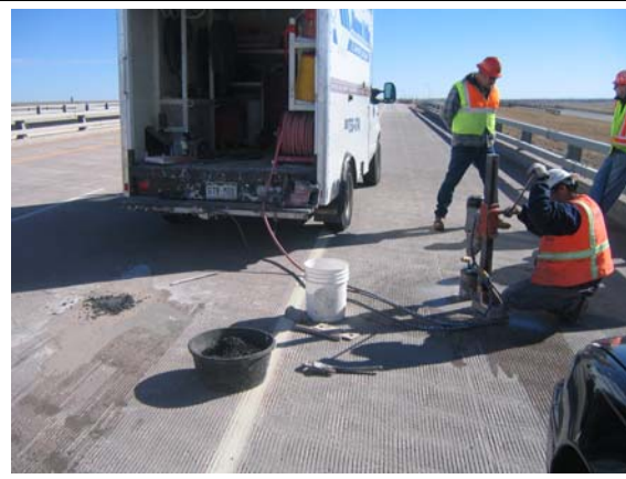
Figure 14 - Coring Concrete Samples on Bridge G-22-BL from the Shoulder
