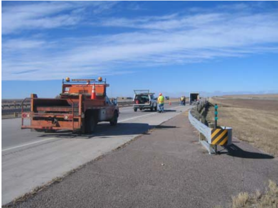
Figure 11 - Bridge G-22-BJ Westbound and CDOT Traffic Control Team
