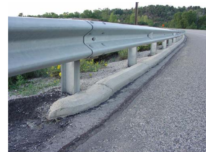
Figure 2. Extruded curb - concrete in this case.
