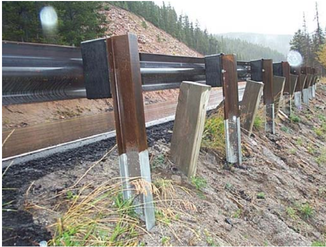
Figure 4. US-50 has steep slopes to both sides.
