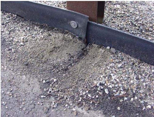
Figure 17. DFC nailed to a guardrail post on US-50.
