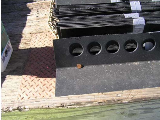
Figure 8. Holes in the horizontal leg of the DFC help the layers of asphalt bond together to strengthen the curb.
