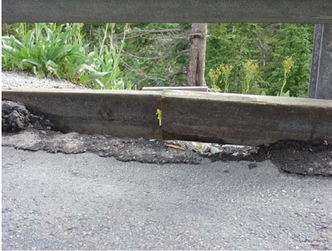
Figure 3. Wood curb can twist and warp.
