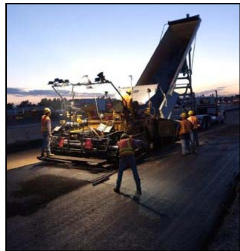
Figure 1. Asphalt Paving Operations on the T-REX Project
