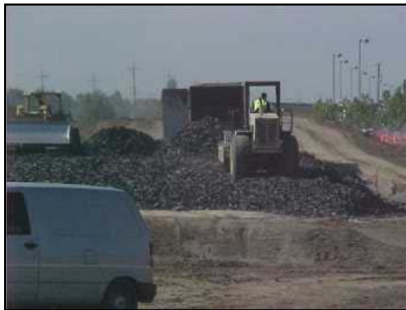
Figure 4. Caltrans Uses Shredded Tires in Highway Embankments
