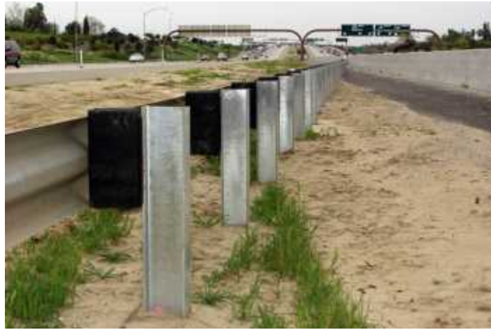
Guardrail can be dismantled and used again.
