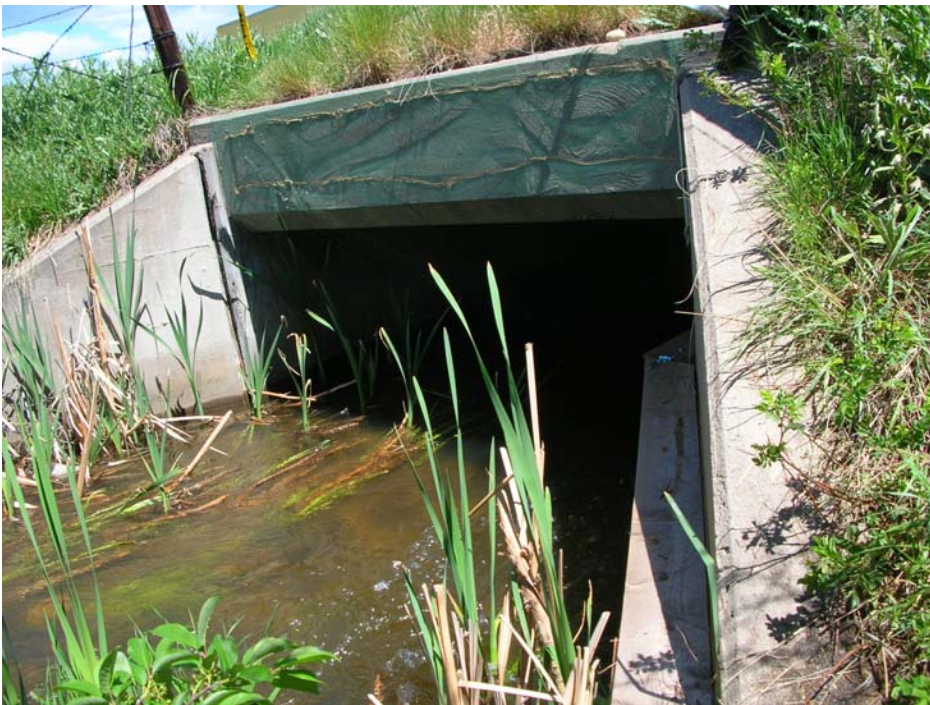
Culvert 2. Marshallville at U.S. 36.
