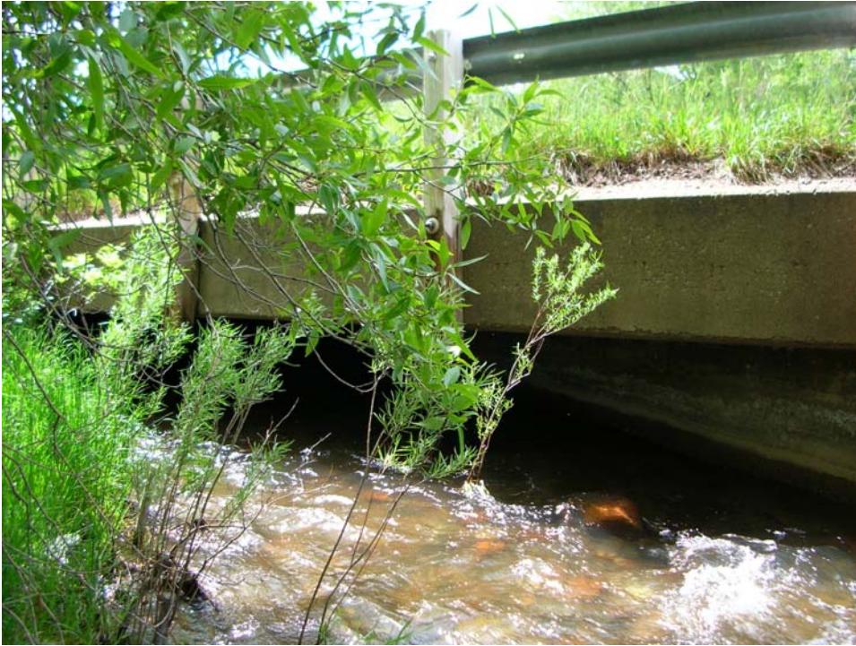
Culvert 7. Davidson Ditch at State Highway 170 in Eldorado Springs.
