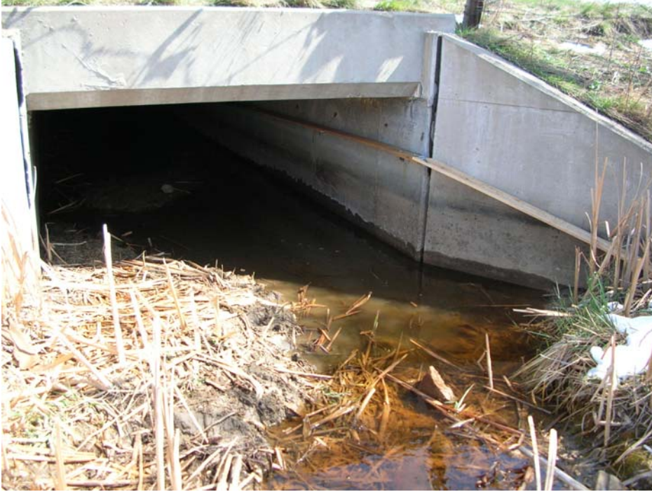
Culvert 1. Dry Creek Ditch No. 2 at U.S. 36.
