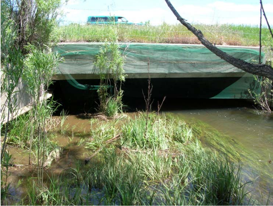
Culvert 3. Goodhue Ditch at U.S. 36. Bird netting visible.
