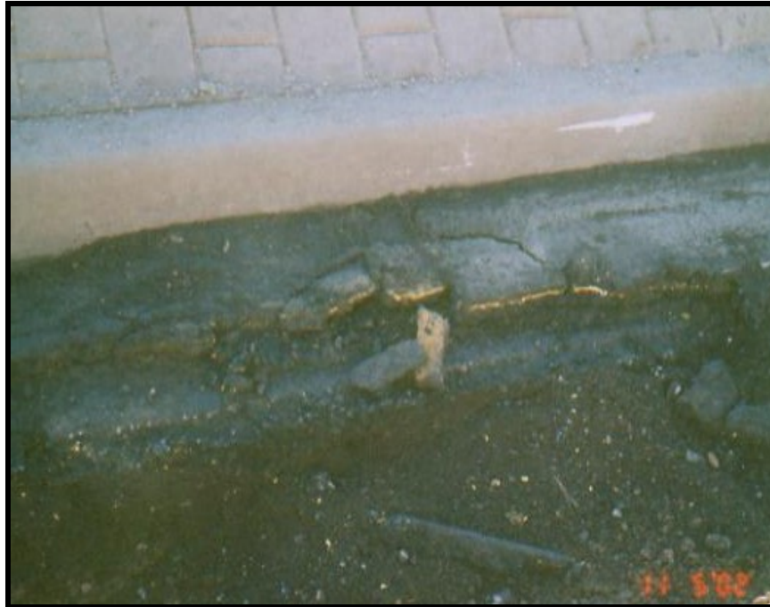
Figure 31: Asphalt removals during rehabilitation construction
