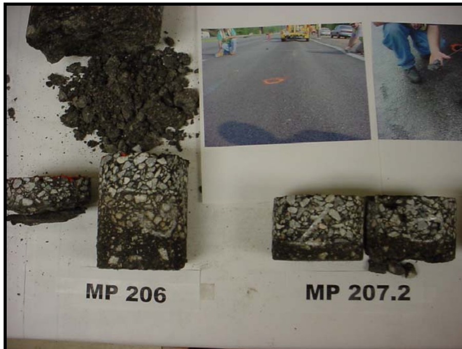
Core samples showing moisture damage and pictures of rutting
