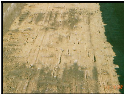
Figure 3: Roadbase exposed during asphalt remediation
