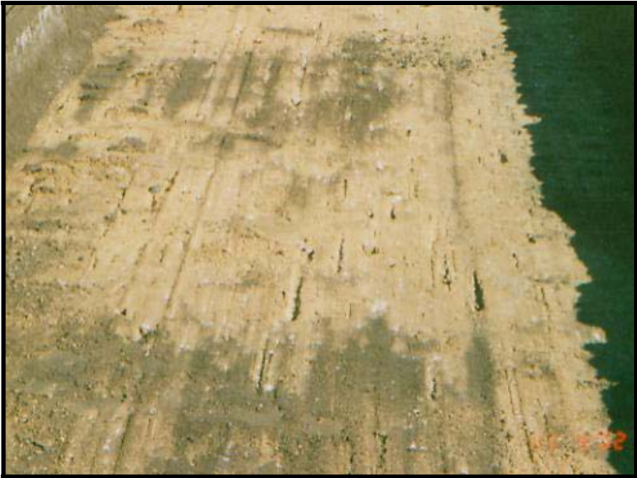
Figure 30: Roadbase exposed during remediation
