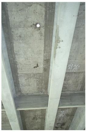
Figure 4.28. Photograph from beneath bridge deck after coring operation.
