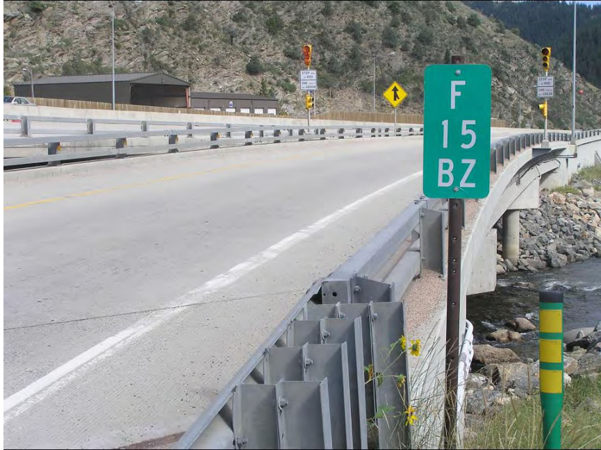
Figure 11. Structure F-15-BZ west of Idaho Springs
