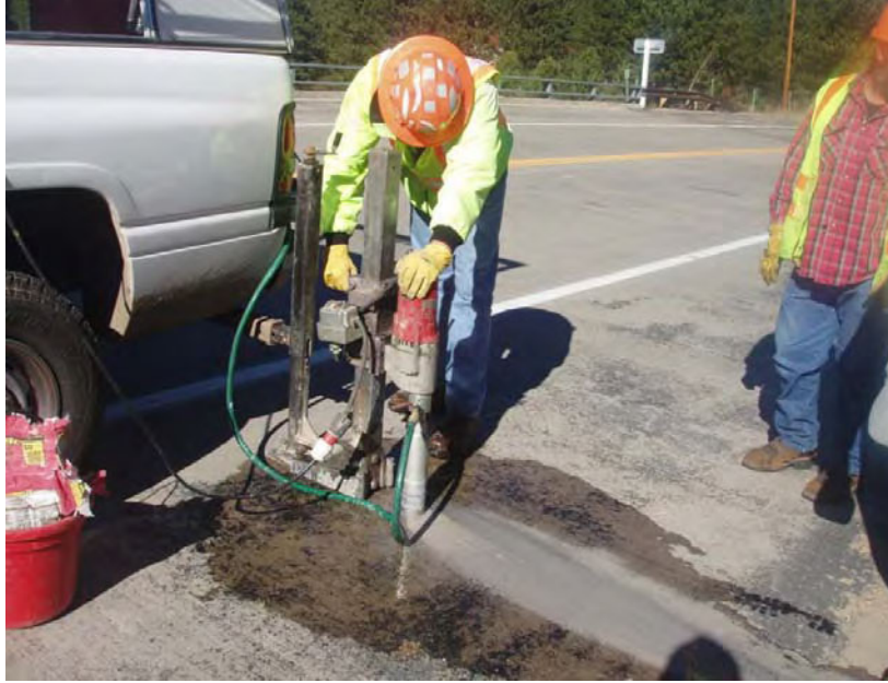
Figure 7. Bridge deck coring
