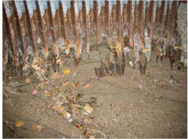
Figure 7. Culvert pipe corrosion near Castle Rock, I-25
