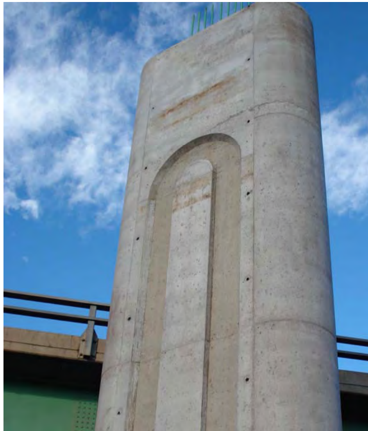
Figure 23: Visible Placement Separations
