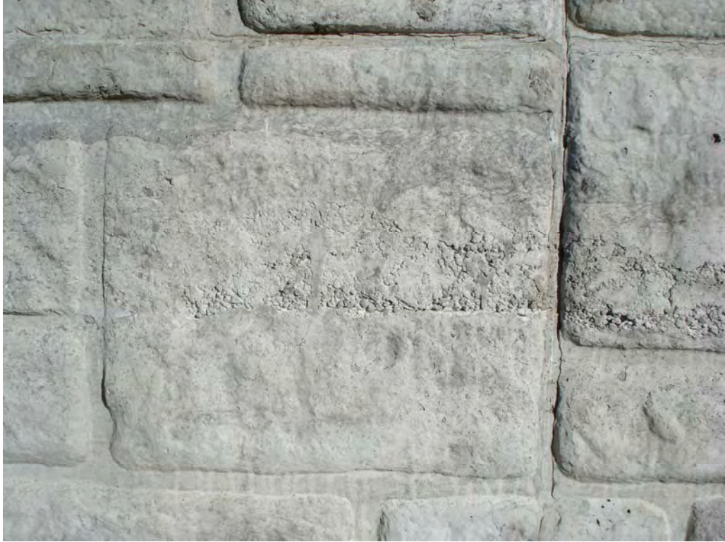
Figure 17: Southern Abutment Finish 1
