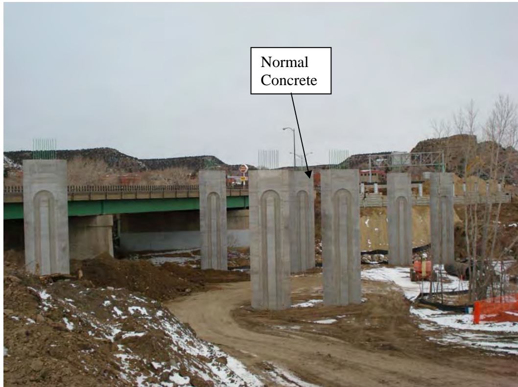
Figure 21: Northbound Bridge Piers
