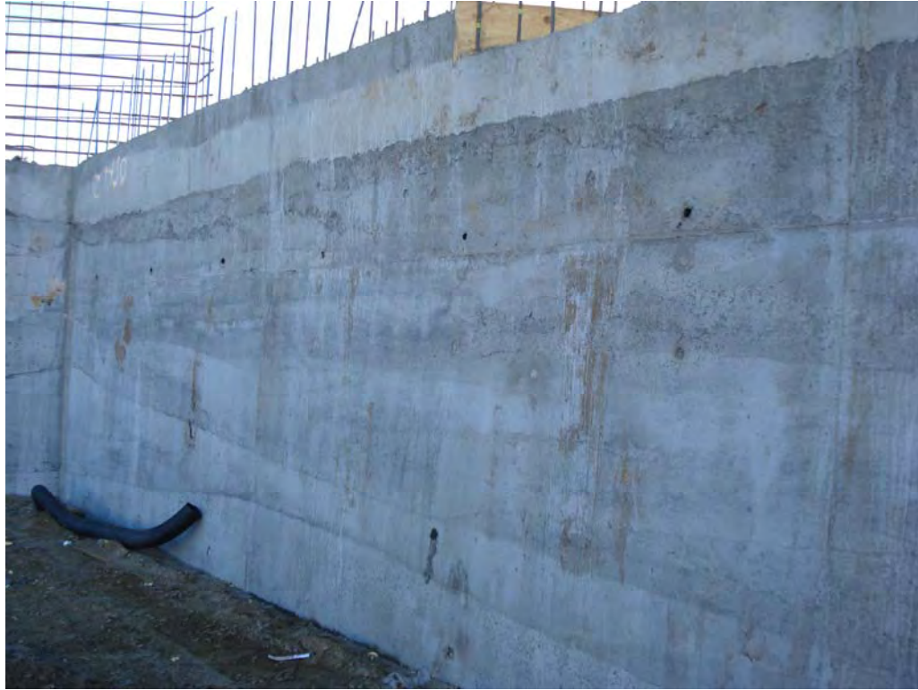
Figure 15: Stratification of SCC
