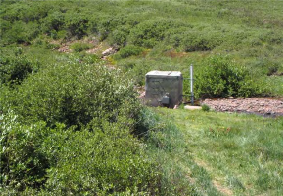
Figure 20. Water Pump From Vail Pass Ten Mile Creek
