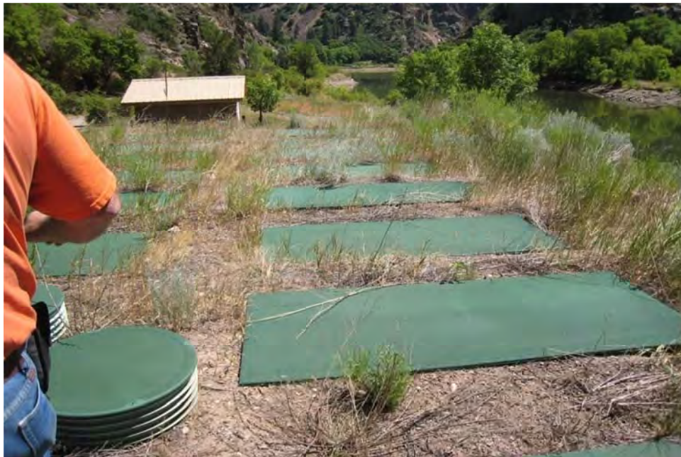
Figure 13. Hanging Lake Rest Area Wastewater Treatment System
