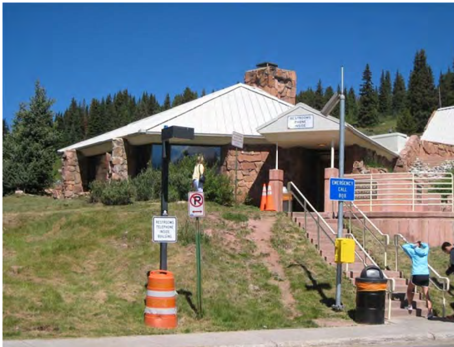
Figure 18. Vail Pass Rest Area Restroom Structure
