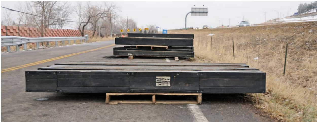
Figure 5. Tire-Ties™ Staged for Construction
