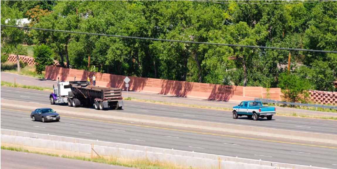
Figure 6. Completed CDOT Barrier Wall from US 6 Side
