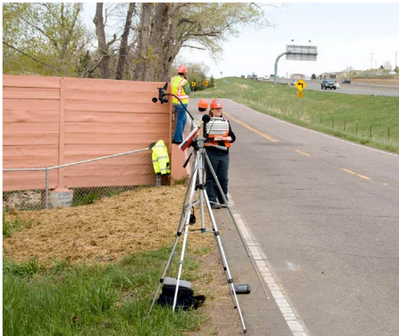
Figure 4. Measurement of Barrier Noise Reduction (Looking East)
