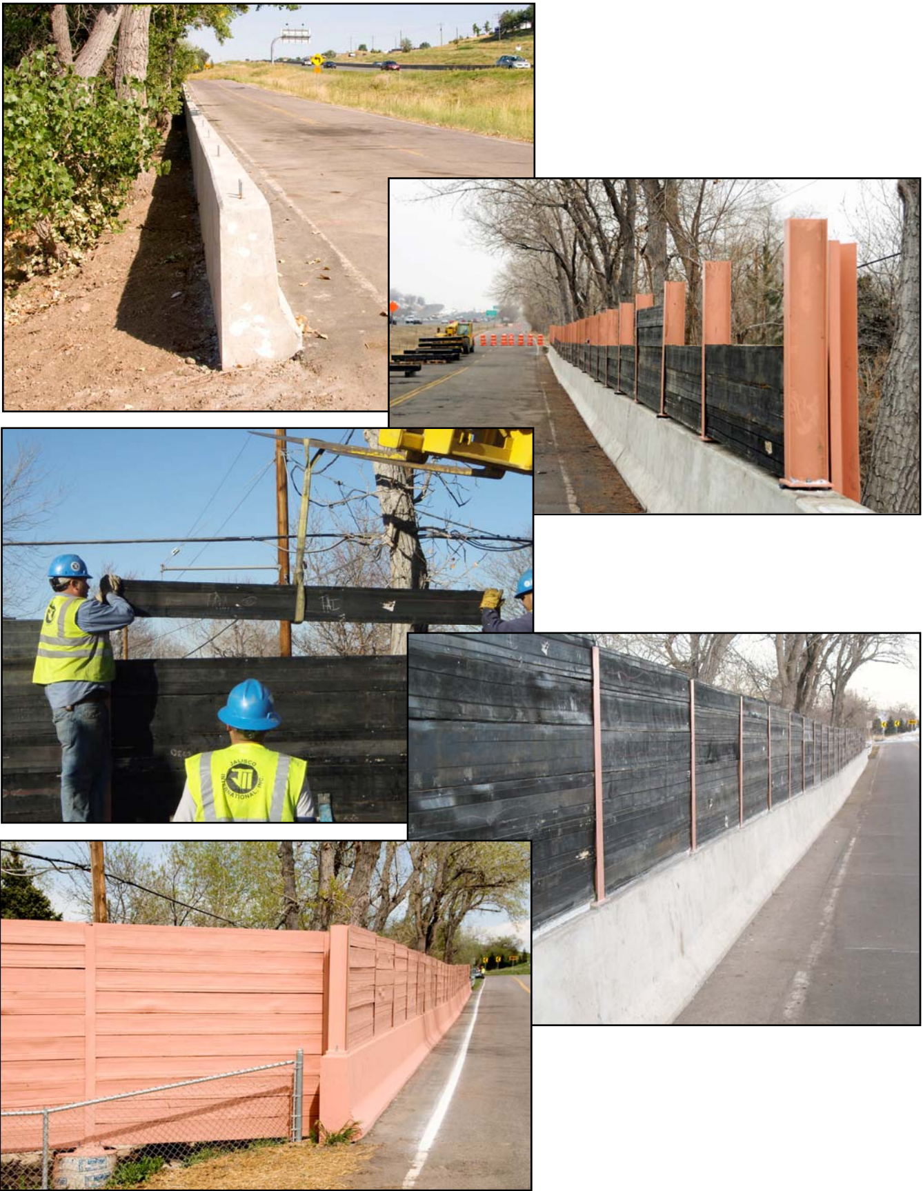
Figure 3. Construction of CDOT Barrier Wall
