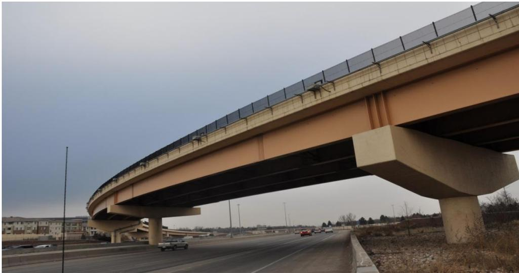
**Figure 4: Long-span bridge with steep cross slope and sharp horizontal curve**
