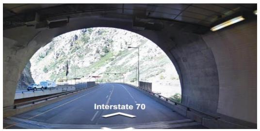
Figure 5: Tunnel exit with a bridge located on a sharp horizontal curve
