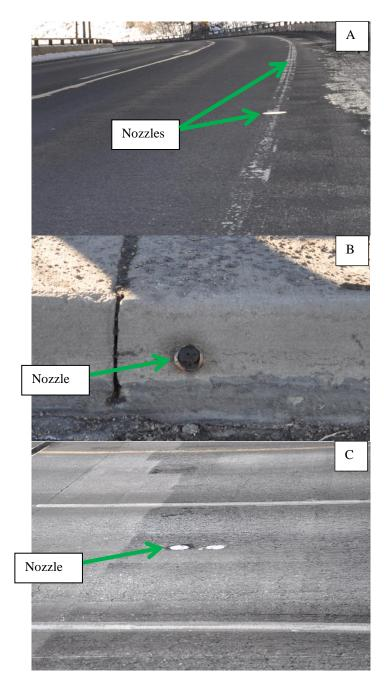
Figure 8: Various locations to mount spray nozzles A) Bridge shoulder B) side rail or side wall C) between two lanes
