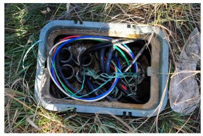
Figure 12: Water leakage in an electrical wiring of a FAST system
