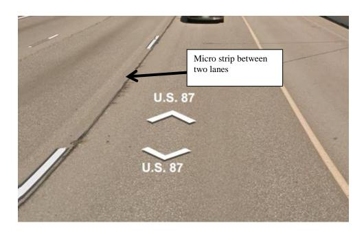
Figure 6: Micro strips on the center of two-lane road
