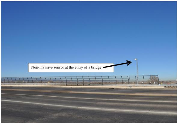
Figure 11: Non-invasive sensors mounted on a pole
