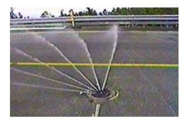
Figure 1: A FAST system in action
