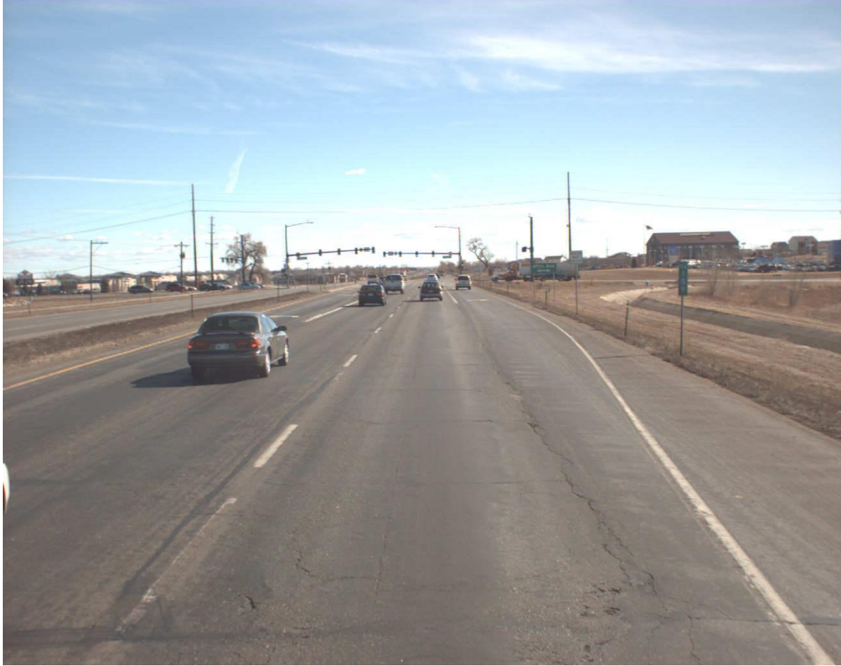
Figure 3. Wet Process Section Looking East
