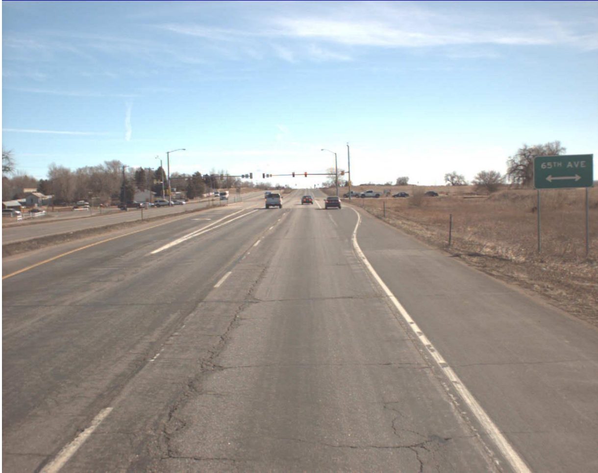
Figure 2. Control Section Looking East
