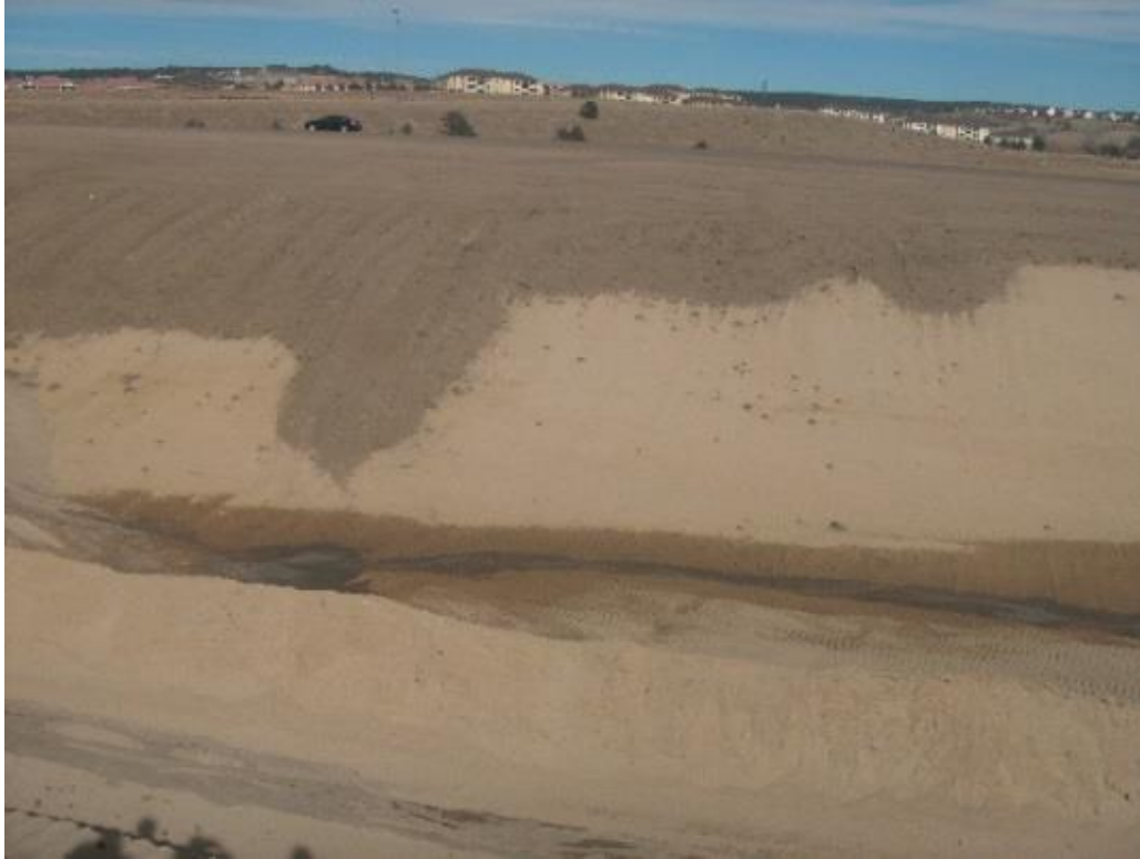
Figure 4. Topsoil spreading in progress.
