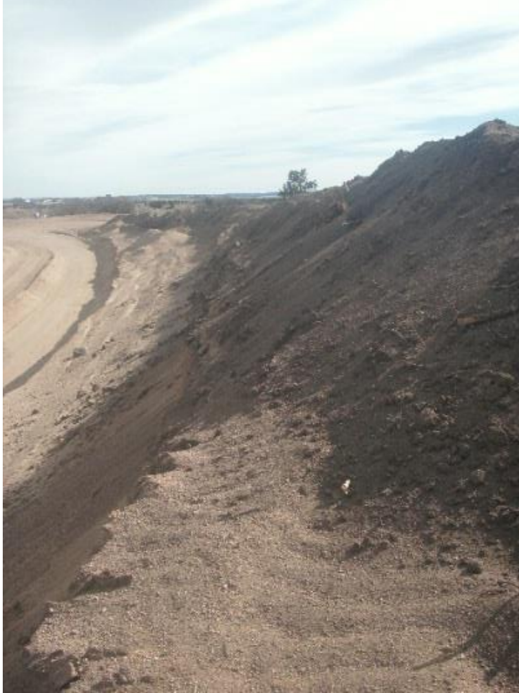
Figure 3. No wind or water erosion control on topsoil piles.
