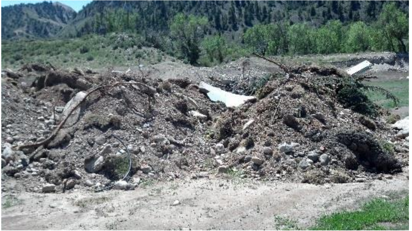
Figure 10. Compromised offsite topsoil stockpile.
