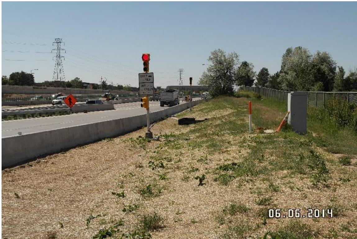
Figure 6. Limited revegetation success due to soil compaction and seed installation
