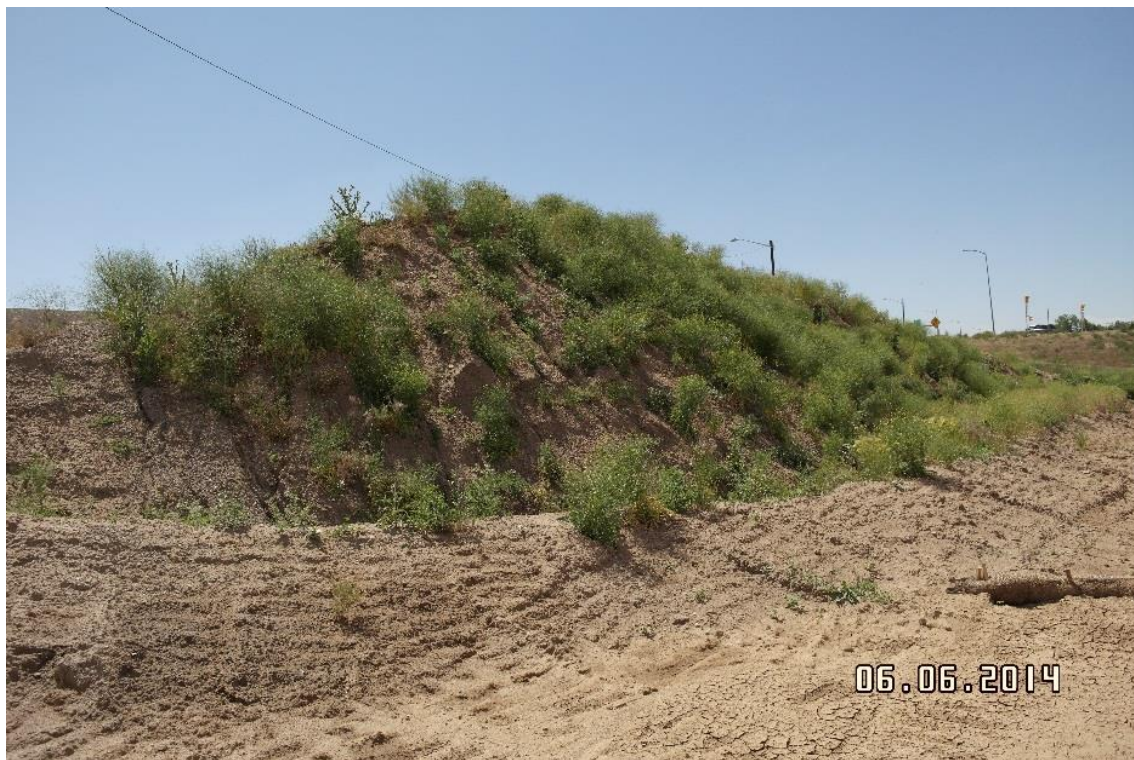
Figure 7. Topsoil stockpile containing noxious weeds and no BMPs.
