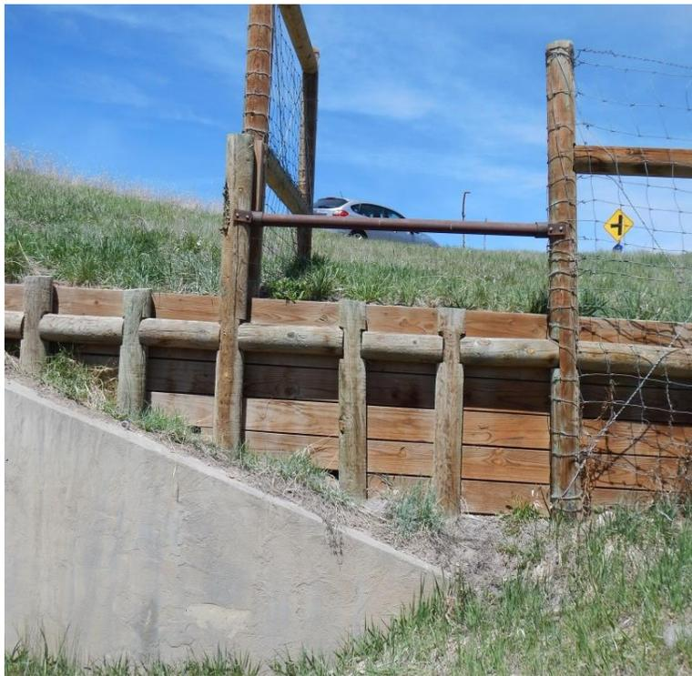
Figure 17. Dry Creek escape jump along Highway 550 from the creek bed.
