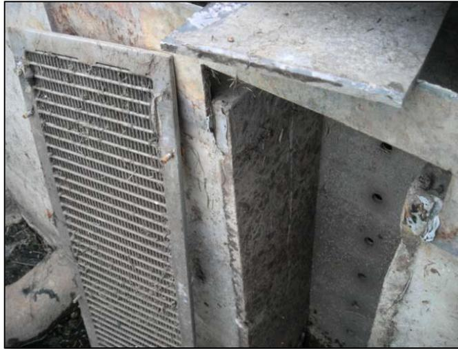
*Figure 1. The current standard for water quality outlet design includes a column of small orifices, protected from clogging by a well screen (shown removed for maintenance). The well screen was added after earlier installations demonstrated a great propensity for clogging. Unfortunately, the well screen also becomes clogged and is considered a significant maintenance issue for CDOT field personnel.*
