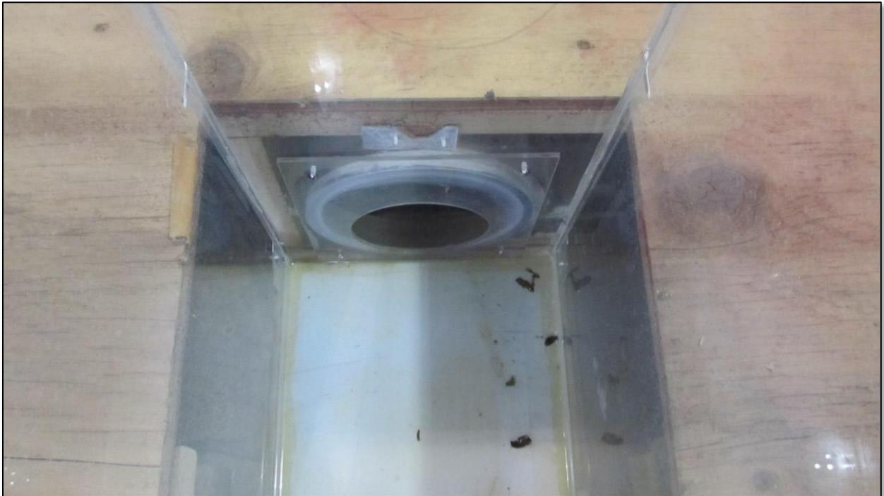
*Figure 40. 100-year restrictor plate covering the final discharge pipe inside the outlet structure.*
