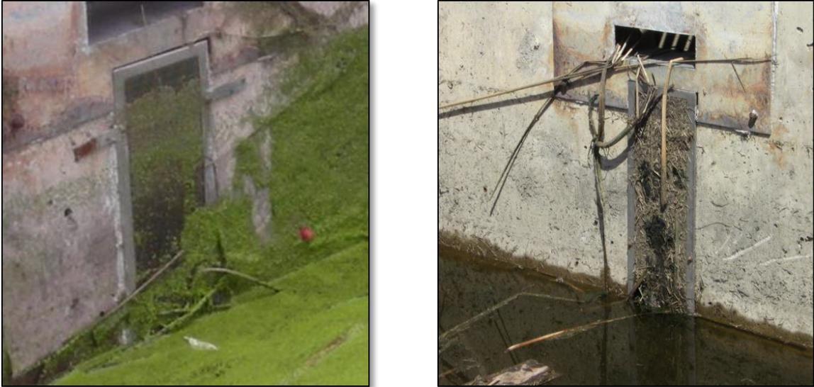
*Figure 22. Typical frequent clogging issues associated with well screens
