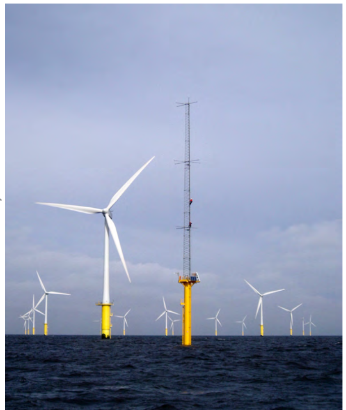
A Campbell Scientific datalogging system monitors this offshore wind farm located between Rhyl and Prestatyn in North Wales at about 7 to 8 km out to sea.
