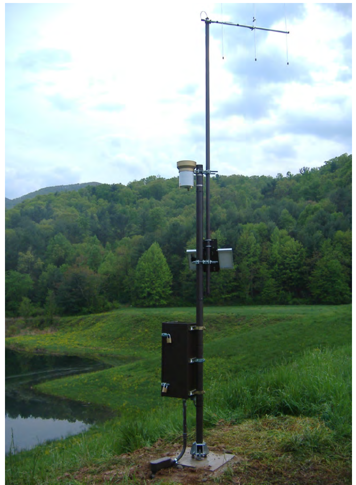
In Virginia, our RF500M Narrowband Radio Modem provides time- and event-driven ALERT data transmission.
