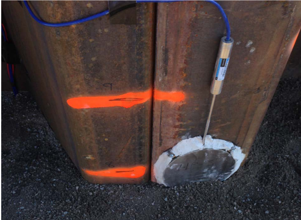
Photograph A-1. Horizontal earth pressure cell install on sheet pile.
