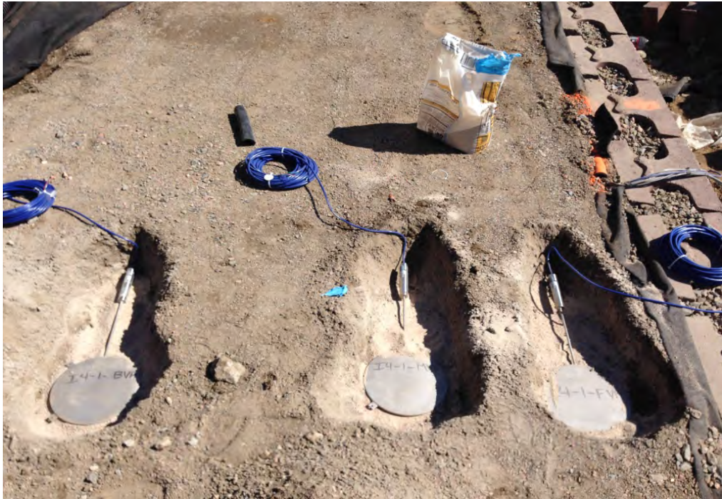
Photograph A-3. Installation of vertical earth pressure cells.
