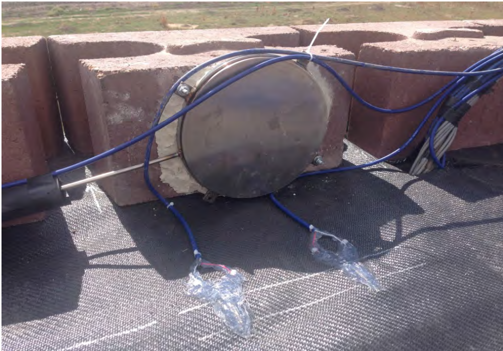
Photograph A-2. Horizontal earth pressure cell install on masonry block.
