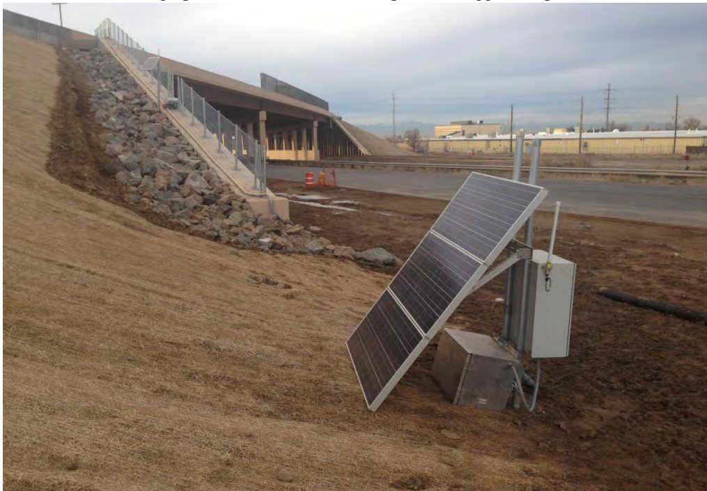
Photograph B-6. Abutment 4 fiber optic data logger.
