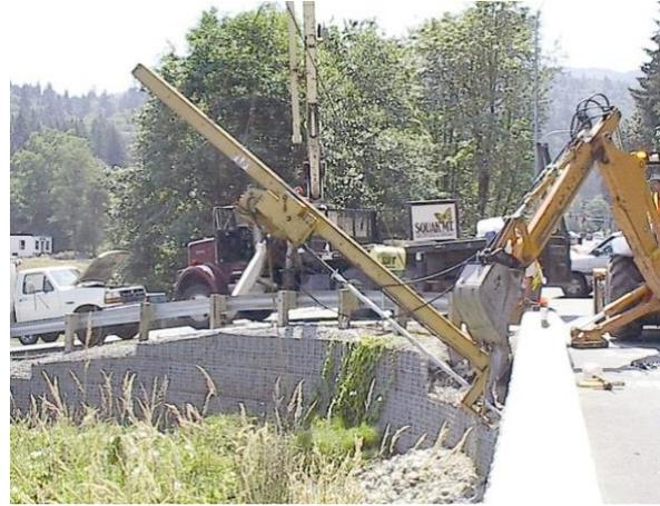
**Figure 1.2: Micropile installation equipment**
