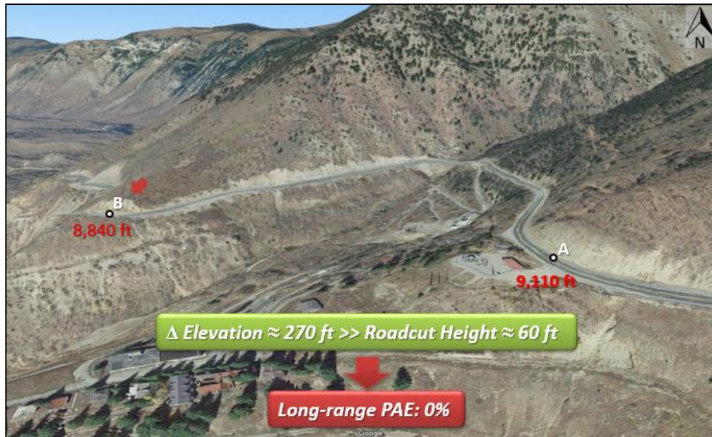
Figure 7. Three dimensional view of HW24 at Vail Pass, Colorado. Note the difference in elevation between the non-adjacent roads and the road cut
