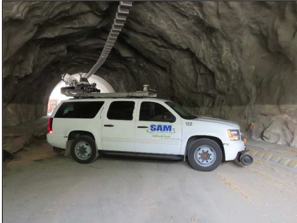
Figure 1: SAM mobile truck in Clear Creek Tunnel #4
