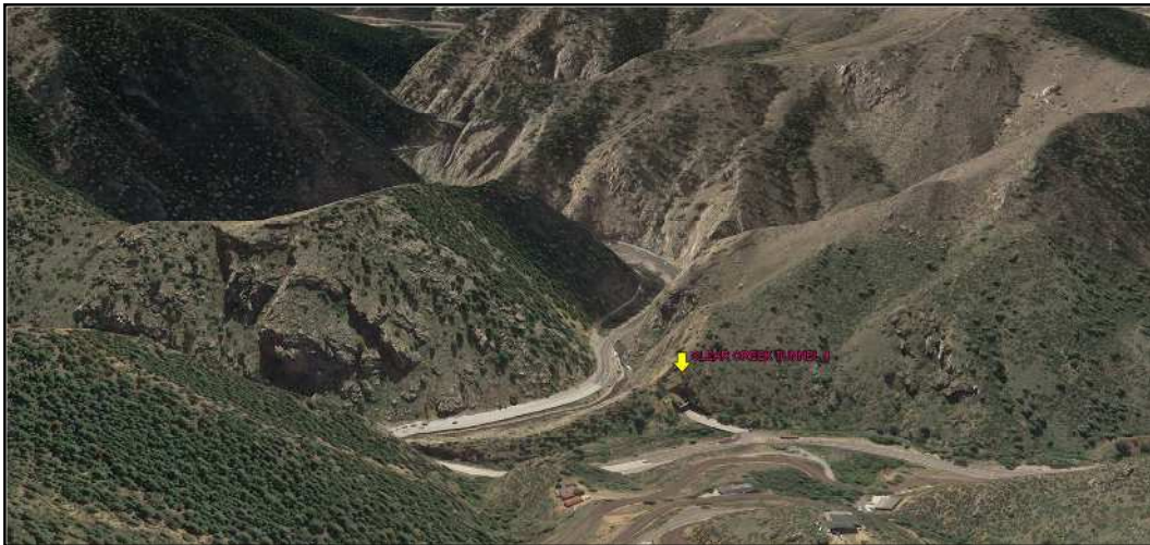
Figure 10: Clear Creek Tunnel 4 aerial
