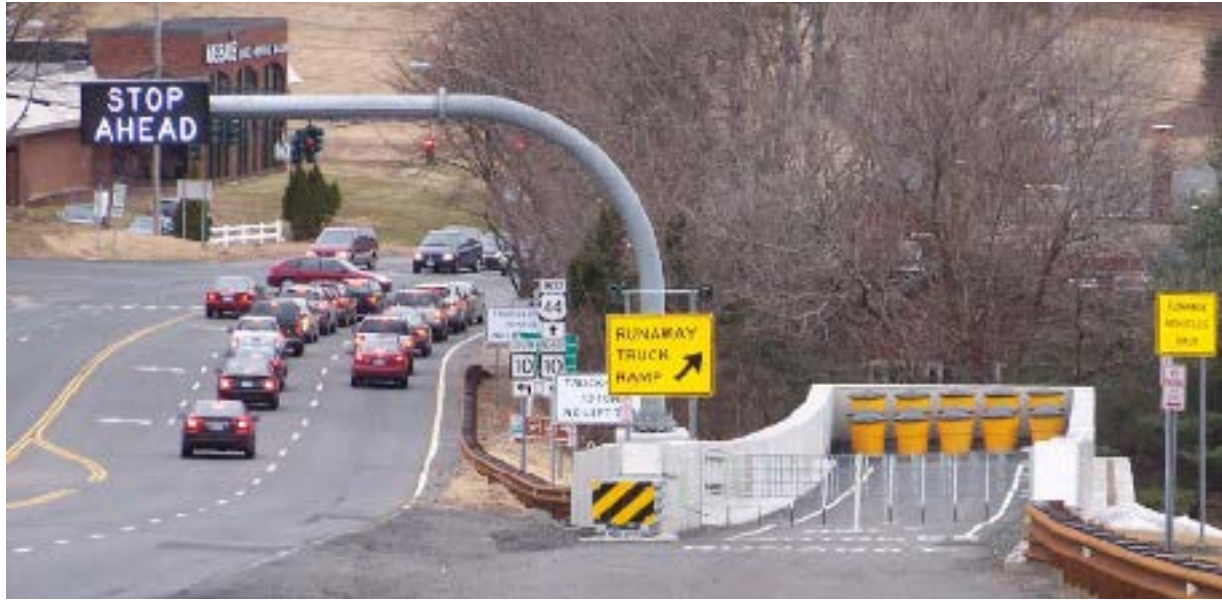
Figure 1.7. Dragnet Arrestor Bed EER with U.44/CT 10/Nod Rd. Intersection in Background Reprinted from Connecticut Department of Transportation's Truck Escape Ramp (TER) (12), 2010, Avon CT.
