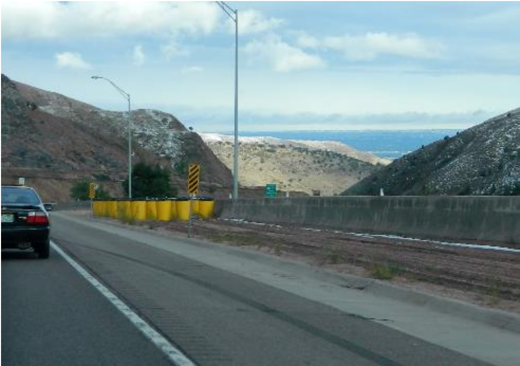
Figure 1.6. Colorado I-70 Eastbound mm 257 horizontal-grade EER
