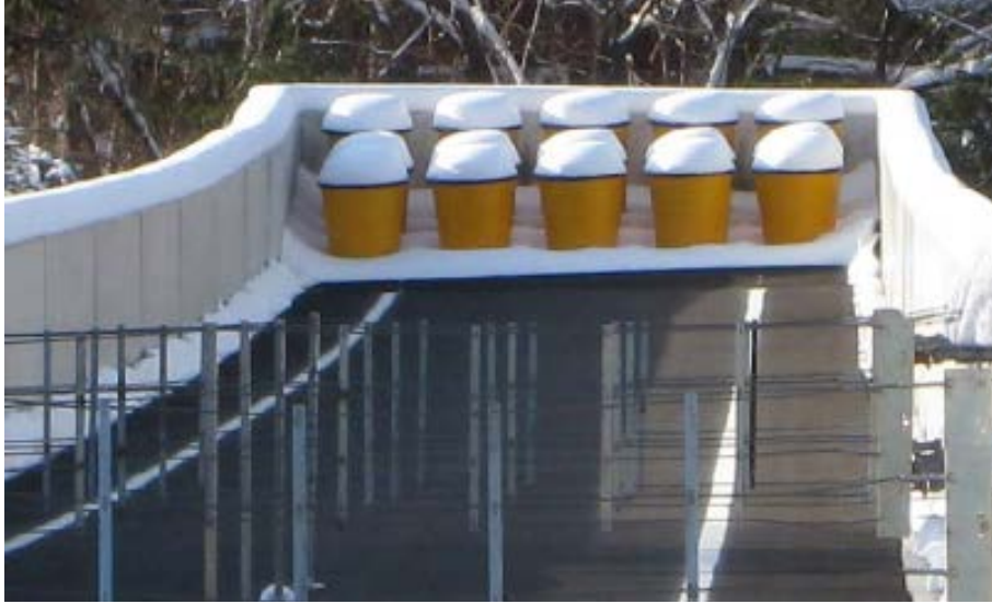
Figure 1.8. Dragnet Arrestor Bed EER after 14” of snow in 72-hour period Reprinted from Connecticut Department of Transportation's Truck Escape Ramp (TER) (13), 2010, Avon CT.
