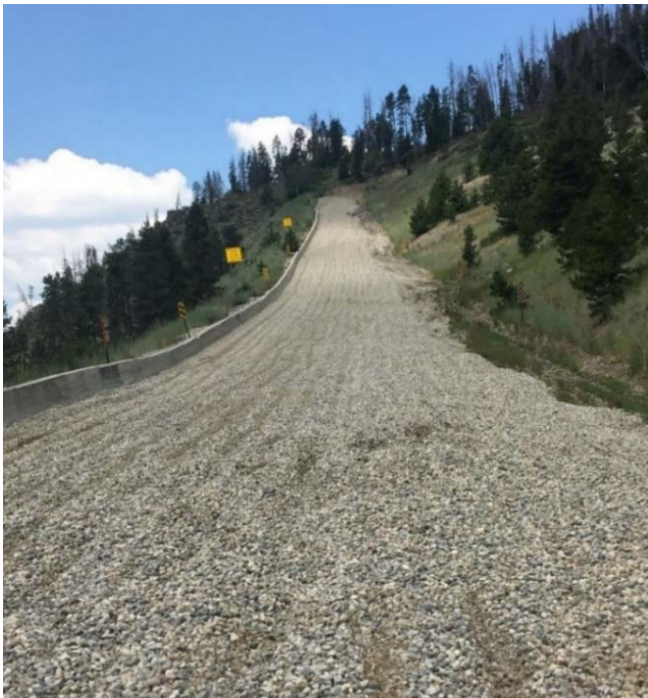
Figure 2.1. The Lower Straight Creek Ramp after Maintenance
