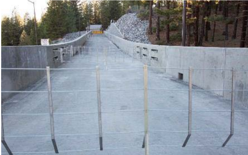
Figure 1.14. The State Route 431 Mt. Rose Highway dragnet EER Nevada Reprinted from Nevada Department of Transportation. Retrieved June 15, 2017, from https://www.nevadadot.com/Home/Components/News/News/90/395?arch=1&cftype=SG0ZO3AZ , Copyright Nevada Department of Transportation, 2016.
