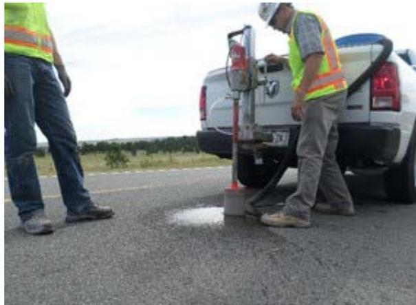
**Figure 82. Coring Operation at SH 86 Kiowa East**
