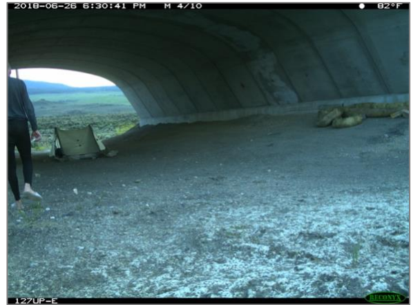
Figure 31. Camper at the Williams Peak Underpass.
