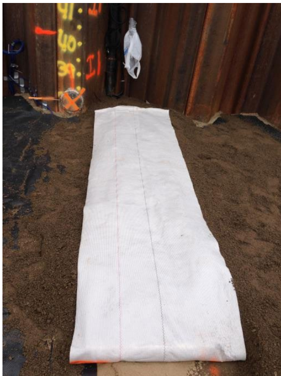
Figure 22. Fiber optic strain gauge field installation
