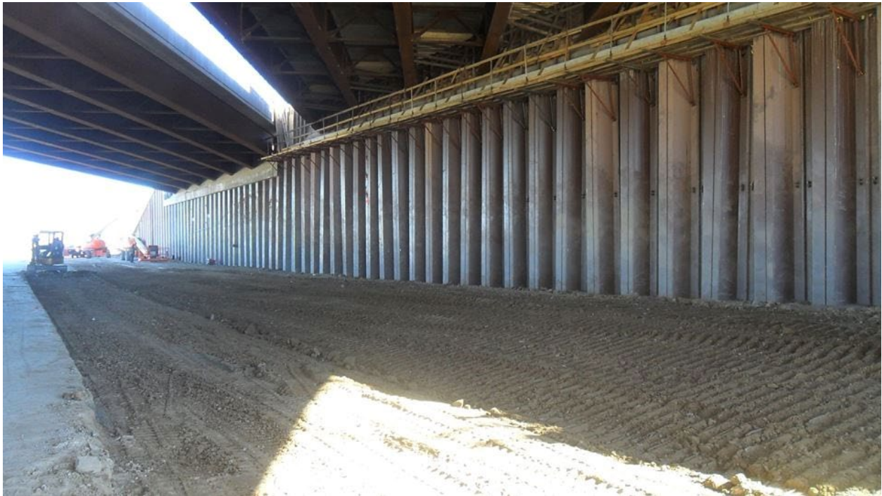
Figure 2. Facing wall of the GRS Abutment #4
