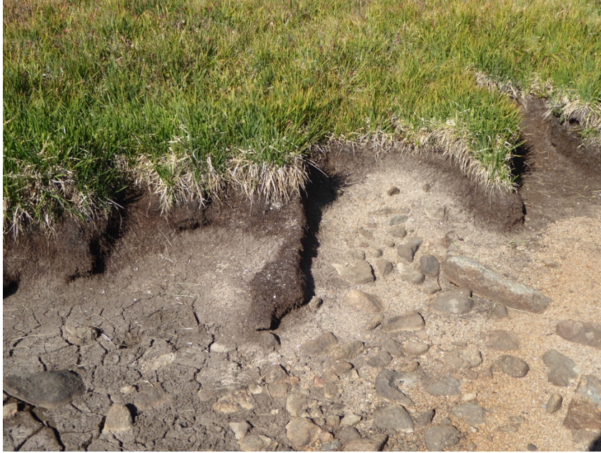
Figure 3. Pool margin erosion illustrated by bare organic rich soils that lack vegetation. Pools appear to be expanding due to erosion.
