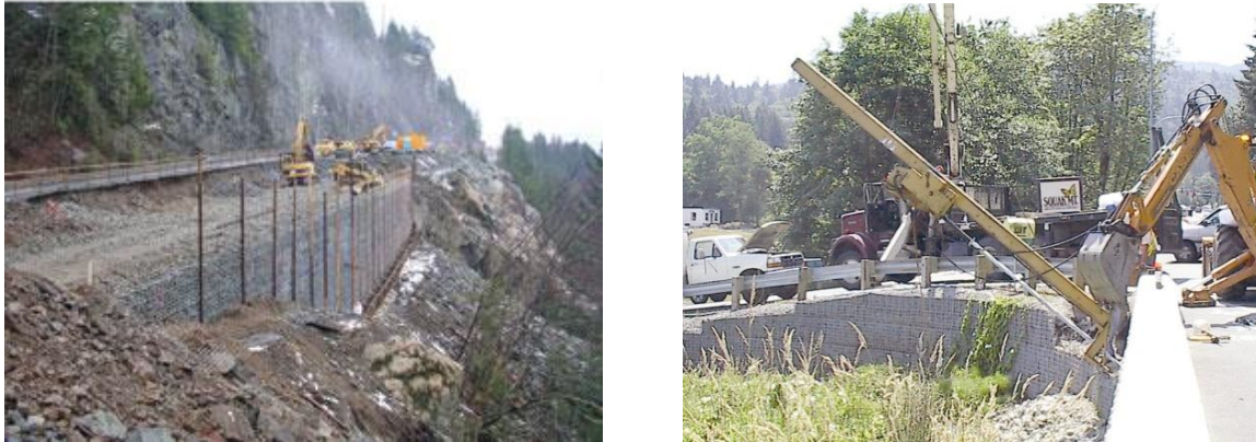
Figure 1.1: Road construction in steep slope and micropile installation equipment
