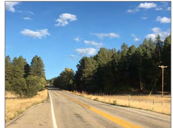
US 84 looking south in this segment
