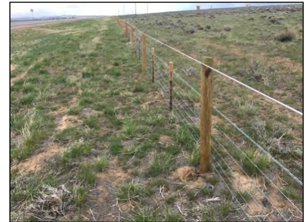
Example of wildlife-friendly sheep fence on State Highway 13 north of this priority segment
