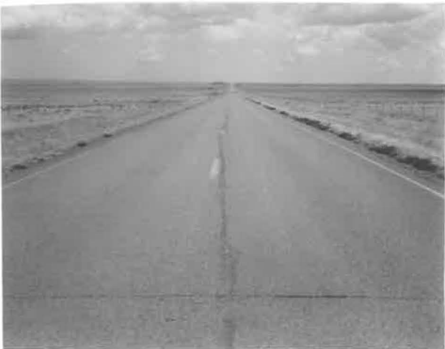
Photograph No. 14 4/28/82 Looking east at Test Sections 5-8 after 4 years. All of the binder materials performed well on this project.
