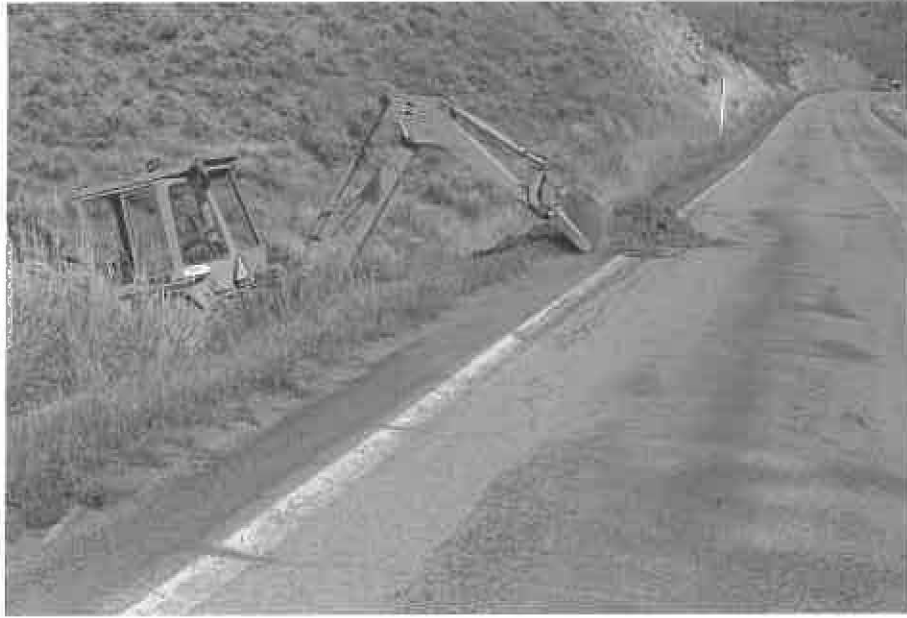
Photograph 2: Using the Department's backhoe, a trench was dug.
