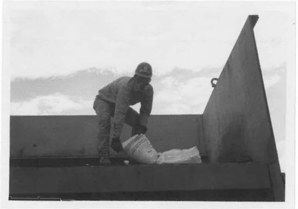
(G) Loading Verglimit into the hopper. Note the use of protective clothing, goggles, and gloves.
