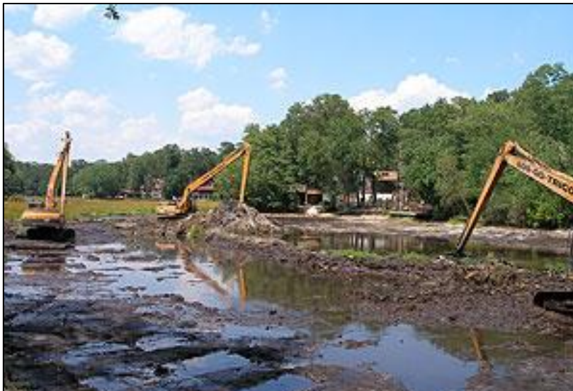
Figure 29: Organic soils being excavated from a project site.
