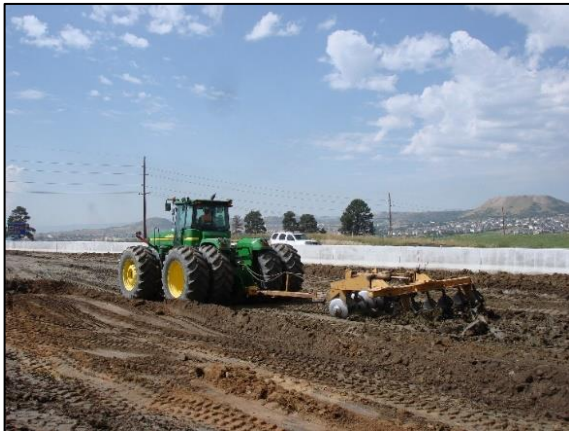
Figure 9: Foundation preparation by means of a tractor with a disk to open the subgrade soils.
