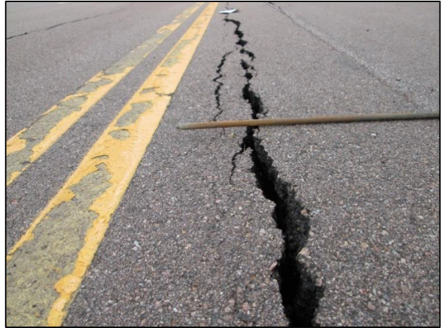
Figure 20: Resultant pavement damage due to differential settlement caused by consolidation of saturated clays beneath a high embankment.
