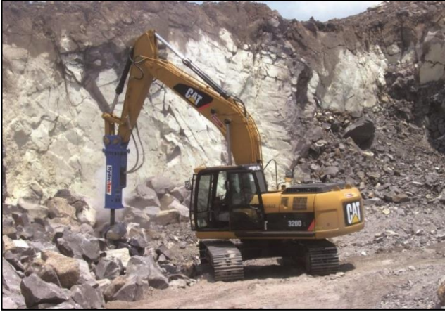
Figure 10: Excavator with hydraulic hammer being used to remove competent bedrock from a cut section.
