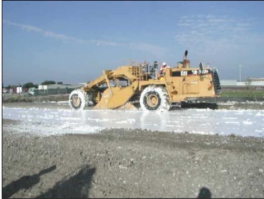
Figure 27: Mixing a lime slurry into subgrade soils to reduce the swell potential.
