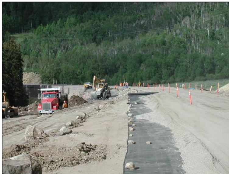
Figure 33: Geotextile installation over soft, unstable subgrade soils
