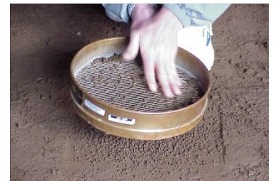
T-310 Figure 6: Filling Surface Voids
