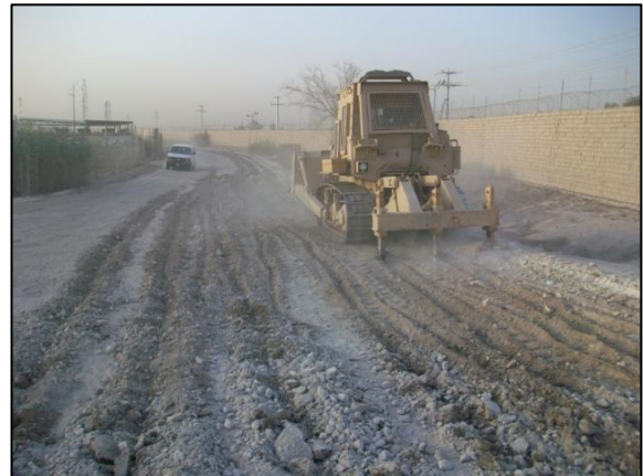
Figure 8: Foundation preparation by means of using a dozer with a ripper attachment.
