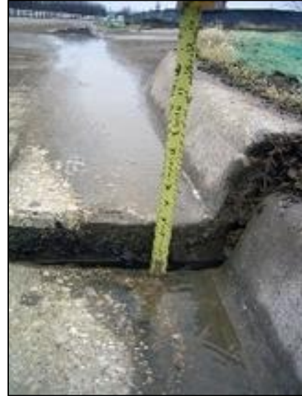
Figure 25: Damage to asphalt pavement and separation along a concrete construction joint as a result of swelling soils.
