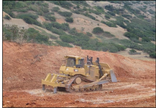
Figure 11: Dozer with ripper attachment being used to loosen material in a cut section.
