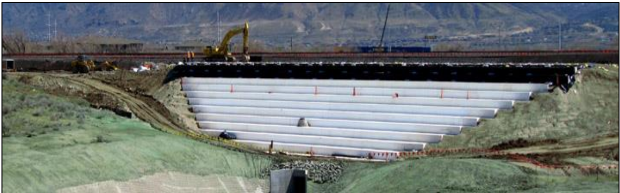
Figure 23: Light-weight EPS foam blocks being used to bridge over soft clay deposits for new embankment construction.
