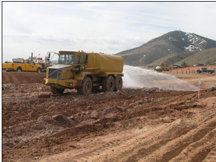
Figure 13: Water truck being used to moisture condition soils in preparation for compaction
