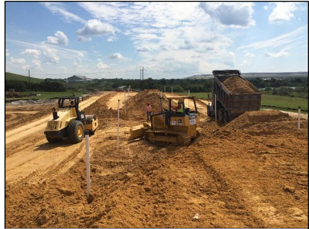
Figure 22: Accelerated consolidation being achieved through the use of surcharging and wick drains.
