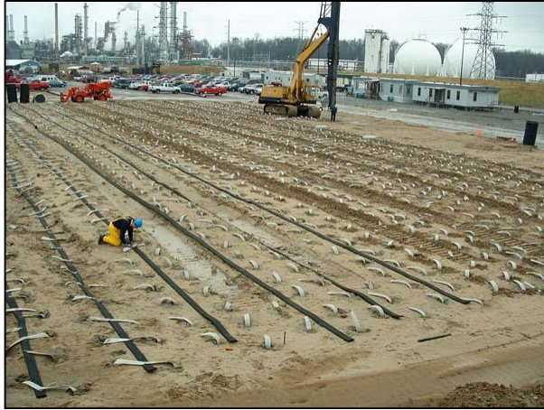
Figure 21: Accelerated consolidation being achieved through the use of surcharging and settlement plates
