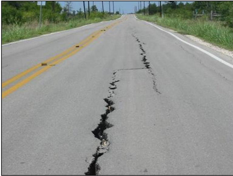
Figure 26: Damage to asphalt pavement and separation along a concrete construction joint as a result of swelling soils.
