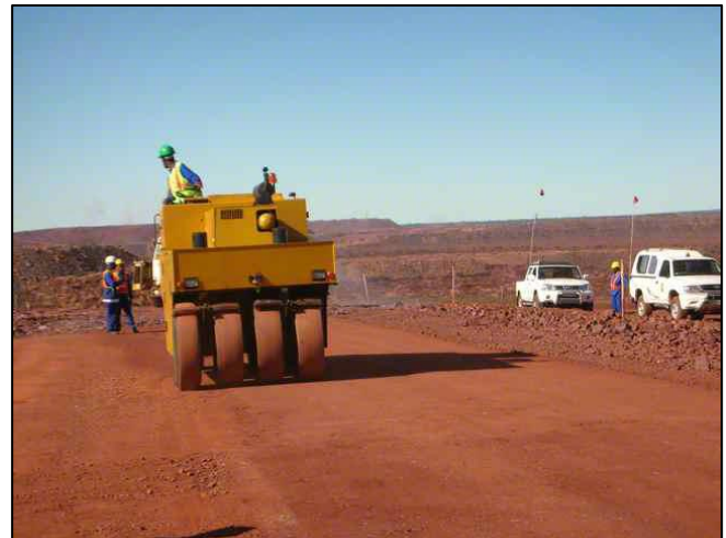
Figure 14: Rubber-tired pneumatic roller
