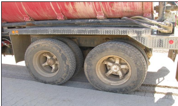
Figure 18: Proof rolling operation being completed by a filled water truck
