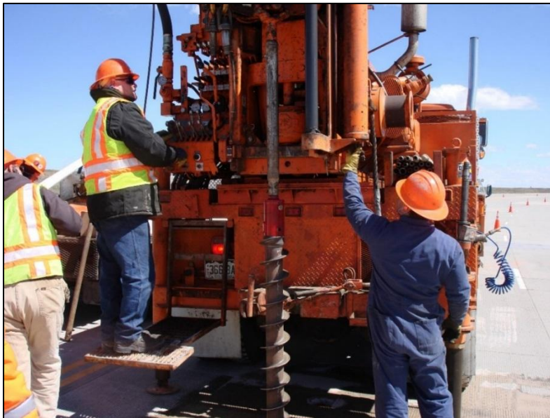
Figure 3: Subsurface explorations and soil sampling being conducted with a drill rig.
