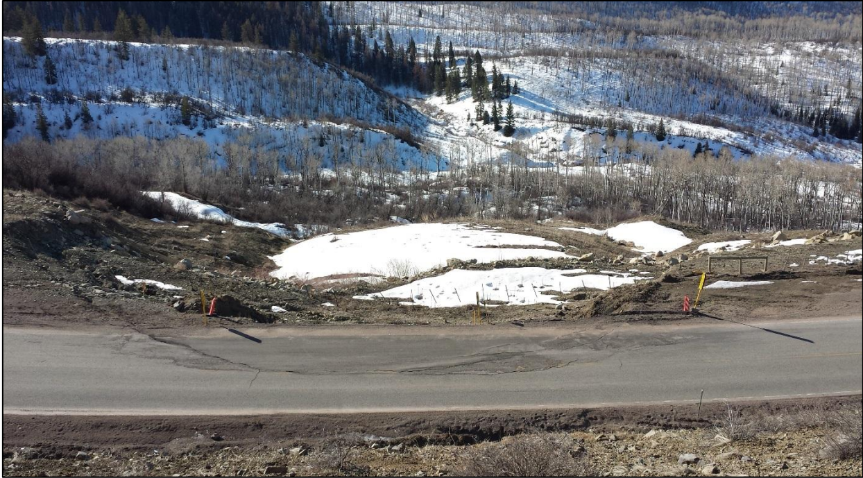
Figure 24: Landslide that developed as a result of embankment construction over a weak clay deposit.
