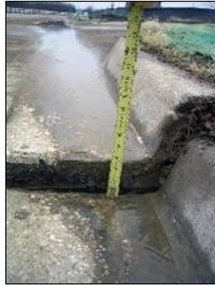
Figure 25: Damage to asphalt pavement and separation along a concrete construction joint as a result of swelling soils.
