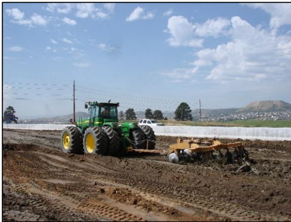
Figure 9: Foundation preparation by means of a tractor with a disk to open the subgrade soils.
