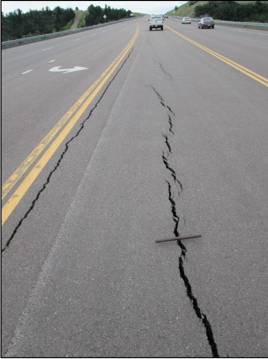
Figure 19: Resultant pavement damage due to differential settlement caused by consolidation of saturated clays beneath a high embankment.
