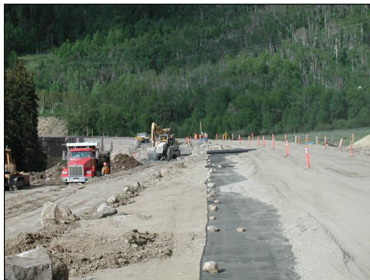
Figure 33: Geotextile installation over soft, unstable subgrade soils
