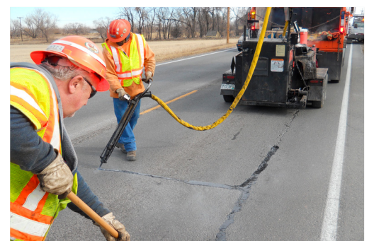
Crew seals cracks on Highway 7 Source: CDOT, 2020
