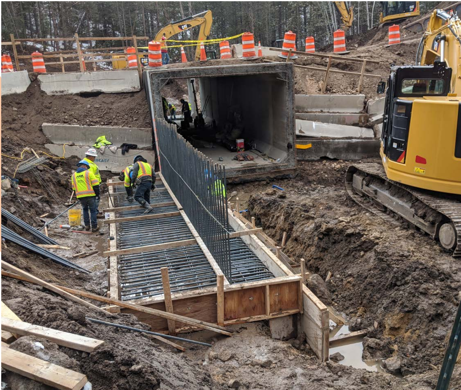
Culvert Install on US 36 near Lion Gulch
