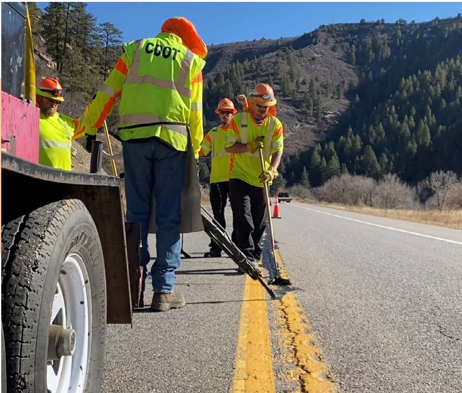
Crack Sealing on US 160
