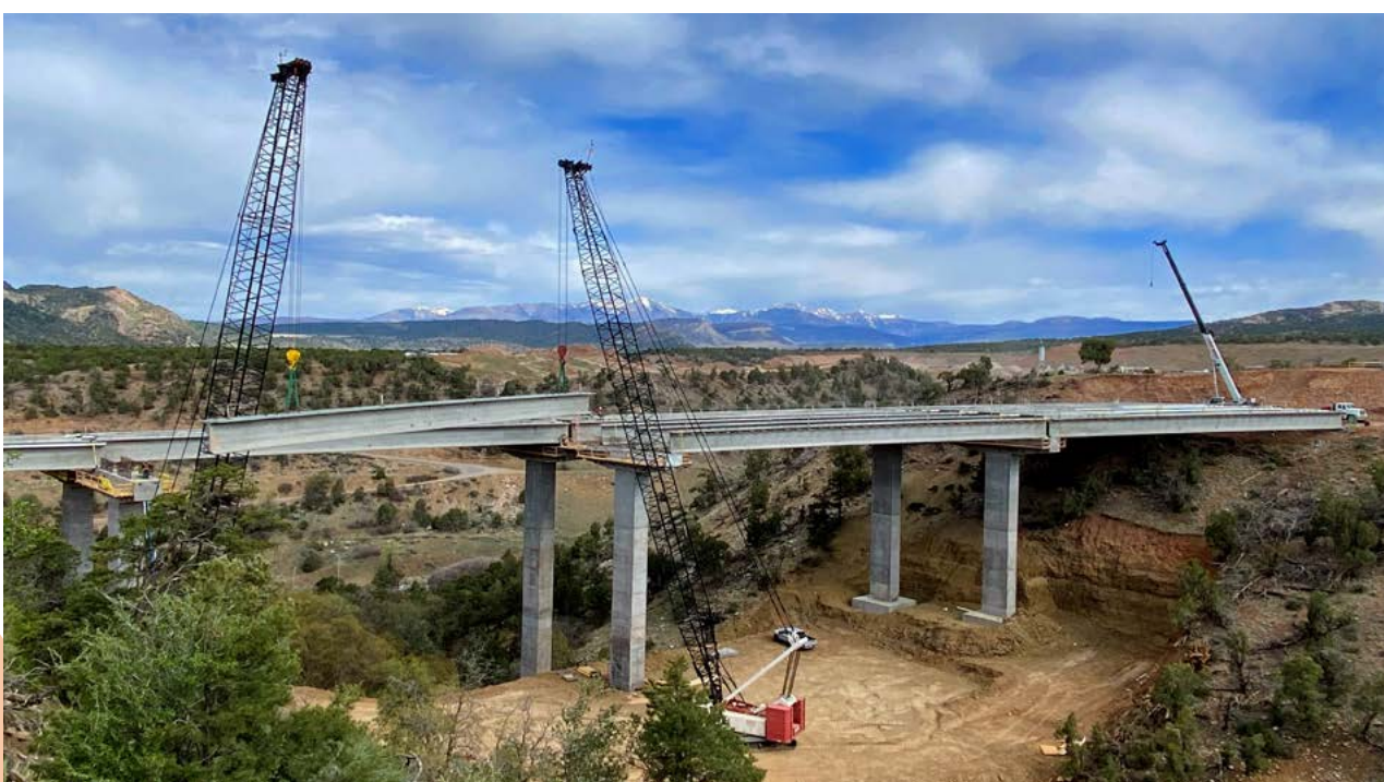
US 550 - US 160 Gulch A Bridge
