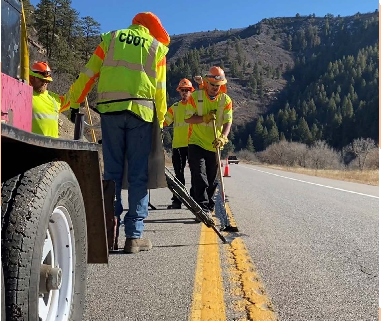
Crack Sealing on US 160
