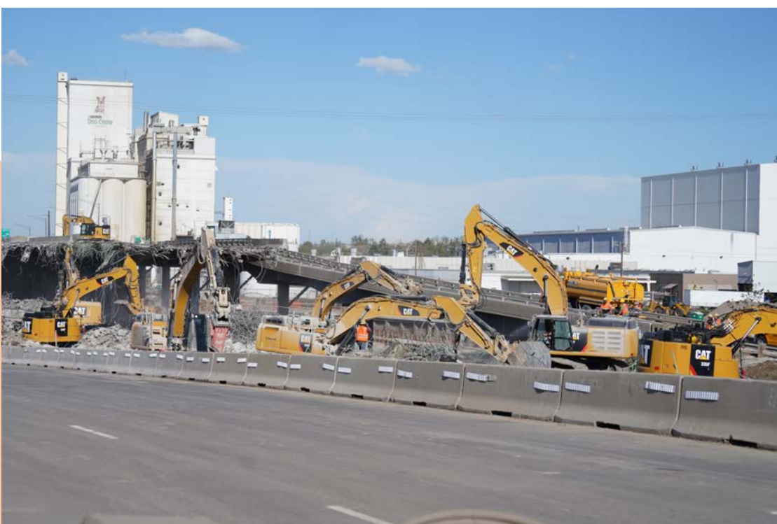
Demolition of Eastbound Lanes
