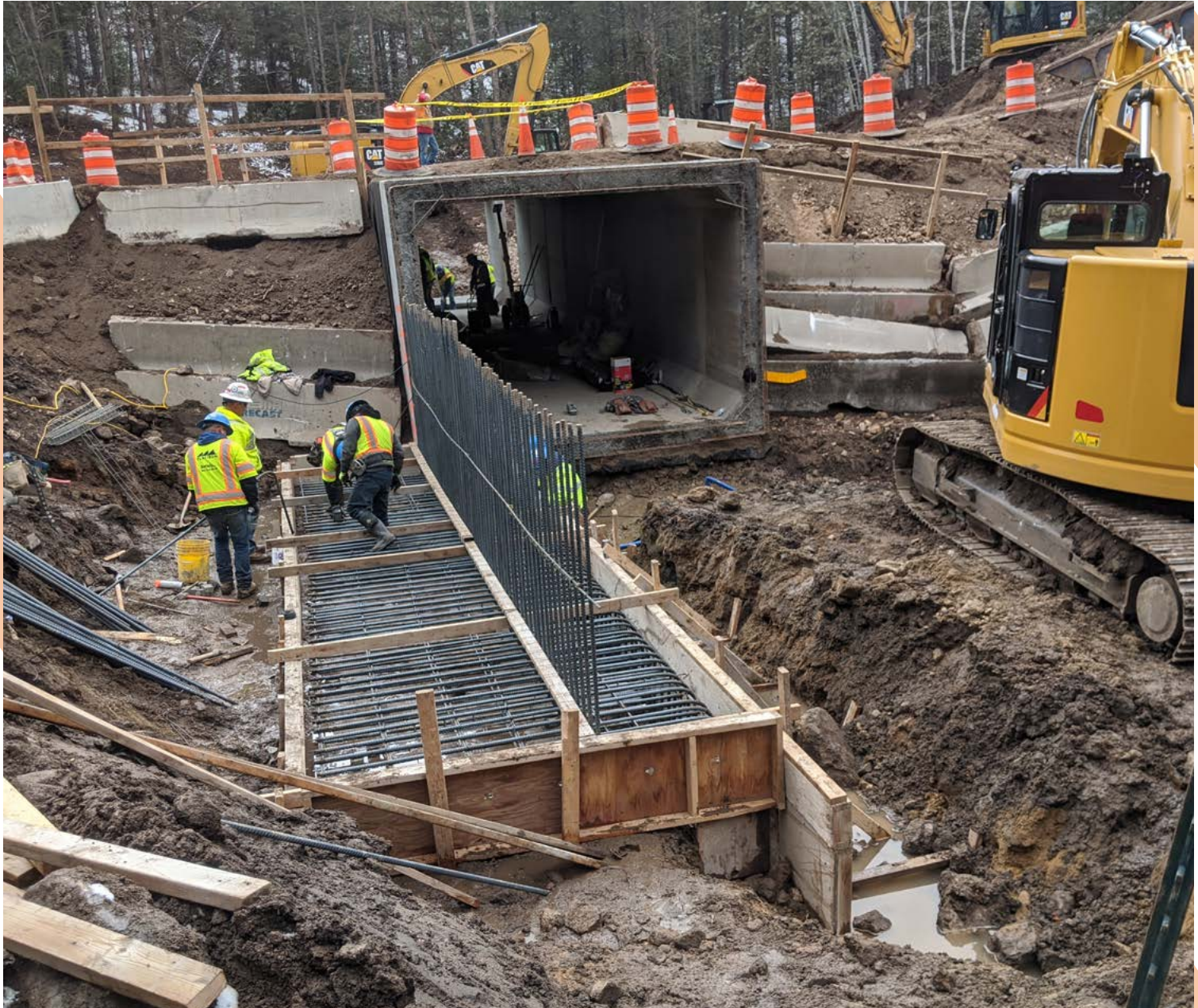
Culvert Install on US 36 near Lion Gulch
